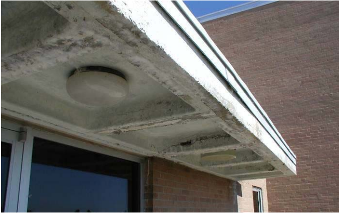
Concrete roof deterioration at the Natural Resources Center – reroofing may have stopped progression of problem.
