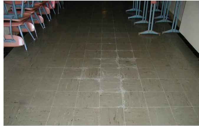
Original vinyl asbestos floor tile deterioration and adhesive failure at Van Lare Hall.
