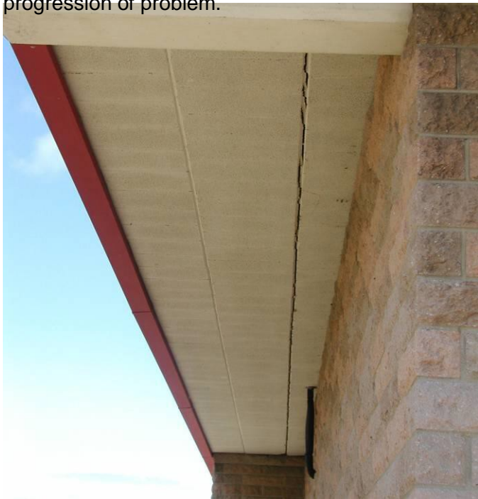
Concrete roof deterioration at the Natural Resources Center – reroofing may have stopped progression of problem.
