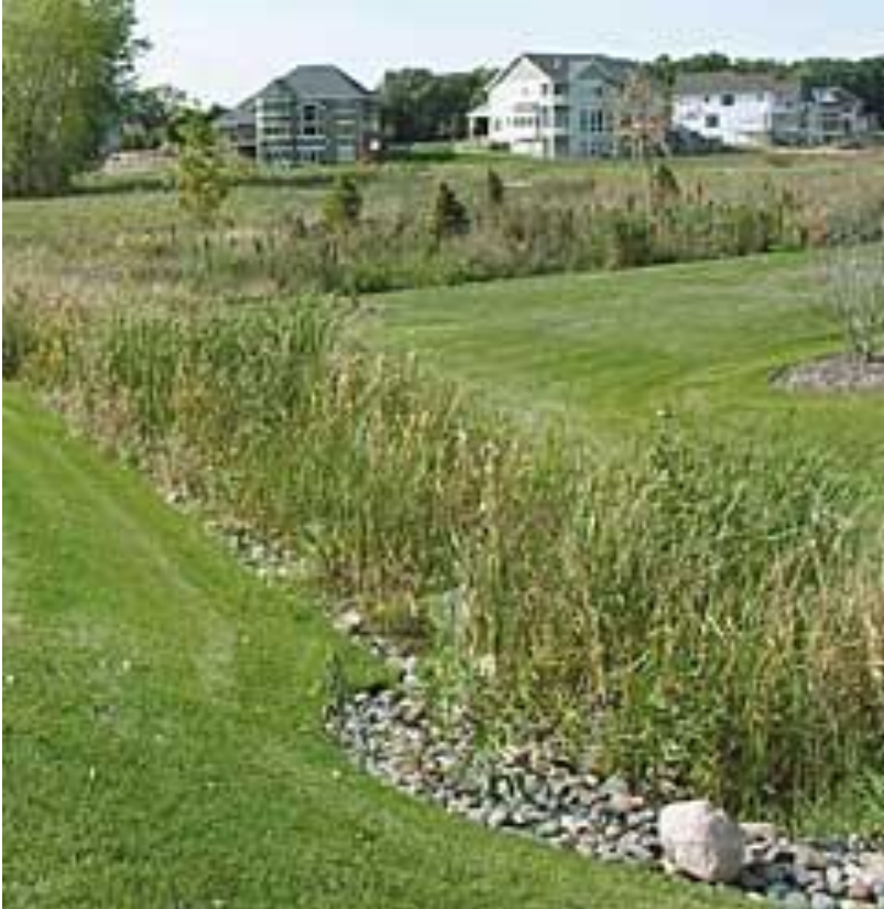
Vegetated drainage along street Showing low impact, sustainable stormwater solutions
