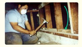
members sit on top of mud sills or cripple walls without blocking between them. The lack of blocking can cause the floor members to fall over sideways in an earthquake. It also makes it difficult to connect the floor to the cripple wall or mud sill. If the blocking is missing between the floor members, it must be added to help put the earthquake forces into the strengthened wall.
