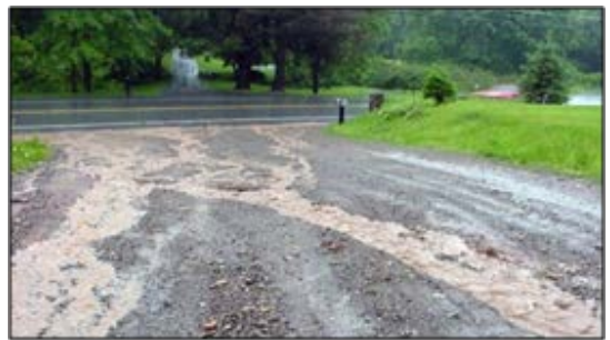
Figure 20. Water in wheel tracks.
