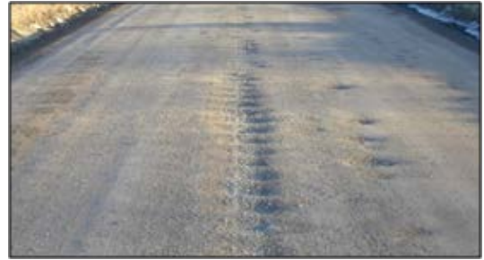
Figure 21. Potholes.
