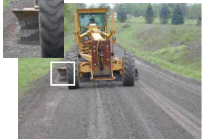
Figure 32. Grader grooming the road. Notice the grader blade is not carrying a lot of material.
