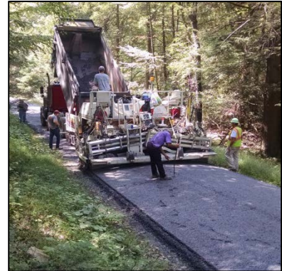
Paver placement of DSA.
