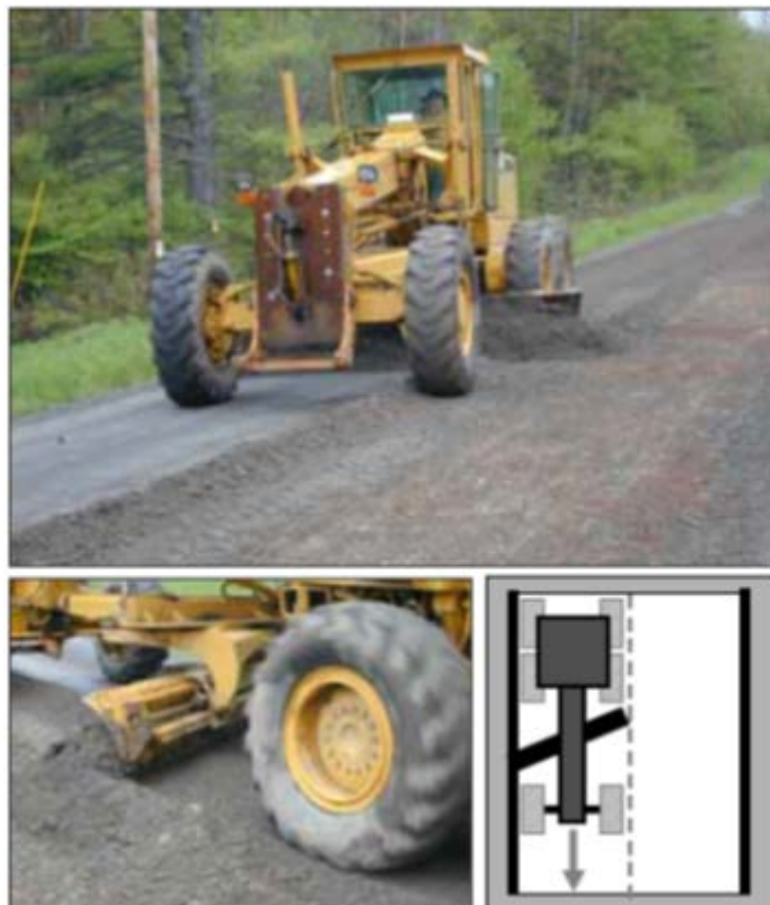
Figure 29. Place grader on one side of crown for each pass.
