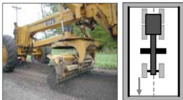
Figure 31. Grader leaving the road with a high flat center.
