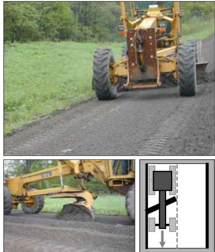
Figure 26. Large aggregate that has accumulated on the shoulder is pulled to the center of the road and mixed with fine aggregate particles as it rides up the blade. The blended aggregate is deposited in a wind-row in the center of the road. Note the high moisture content of the graded material.
