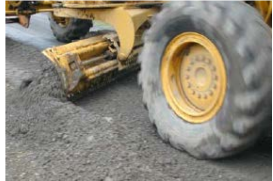
Figure 25: Wet material rolling off blade.
