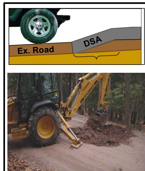
Figure 11. Key cut lengthwise along road prior to DSA placement
