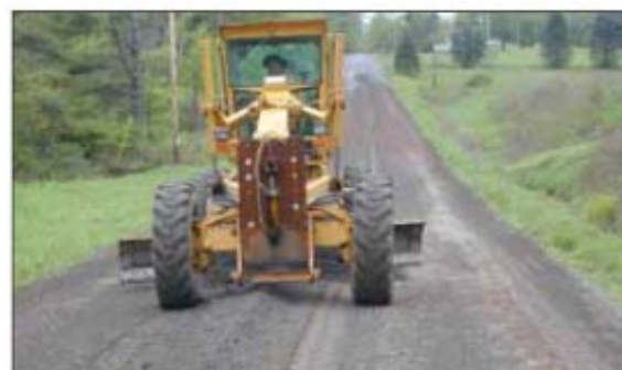
Figure 30. Material is knocked down
