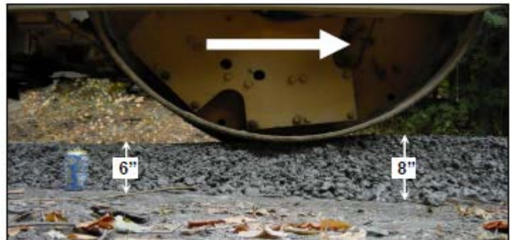
Figure 16. A roller moving from left to right compacts the 8” lift of loose DSA down to 6”.
