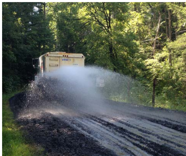
Figure 28. Adding water to a dry road surface.
