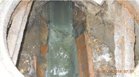
b) Meter #2 collected data during the entire flow monitoring timeframe from 9-7 to 12-4-18. The flow level during low flows at this meter was about 1.5 inch deep and a maximum of 6.6 inches deep during high flows. The velocity at this site was ideal for flow monitoring - ranging from 0.7 f/s during low flow to a maximum of 2.1 f/s during the highest recorded flow.
