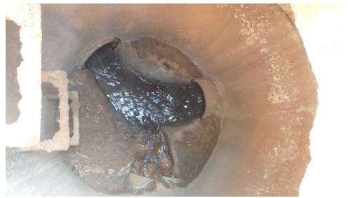
b) Meter #4 was located just downstream of a lift station discharge pipe which cycled frequently and may have affected accuracy. The flow level during low flows at this meter was about 2.1 inch deep minimum and a maximum of 5.5 inches deep was recorded on 10/10/18. The velocity at this site was ideal for flow monitoring - ranging from a low of 0.7 f/s to a maximum of 2.95 f/s during the highest recorded flow on 10/10/18.
