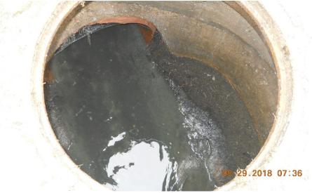
b) Meter #1 collected data from 9-14 thru 12-4-18, on 9-19 the sensor was placed with an offset from the bottom due to silt buildup. The flow level with offset sensor during low flows at this meter was about 1.5 inches deep and the highest level recorded was 13.1 inches deep. The velocity in the pipe ranged from 0.70 f/s during low flows to 1.74 f/s during high flows.
