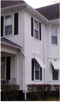
Inconspicuously placed downspouts
