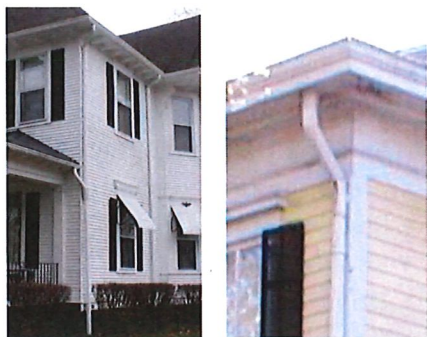
Inconspicuously placed downspouts
