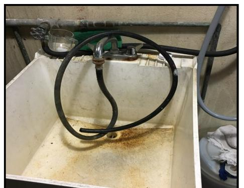
A mop/cleaning sink is present in many homes and businesses. If a hose bibb vacuum breaker is not installed on the faucet, the mucky water in the sink could end up in your potable water system.
