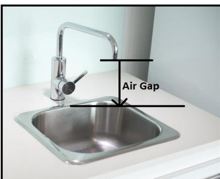
Air gap—the area between the top of the filled container and the bottom of the faucet.
