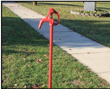
Yard hydrant—these should have at least a vacuum breaker if not Reduced Pressure backflow device to prevent backflow.
