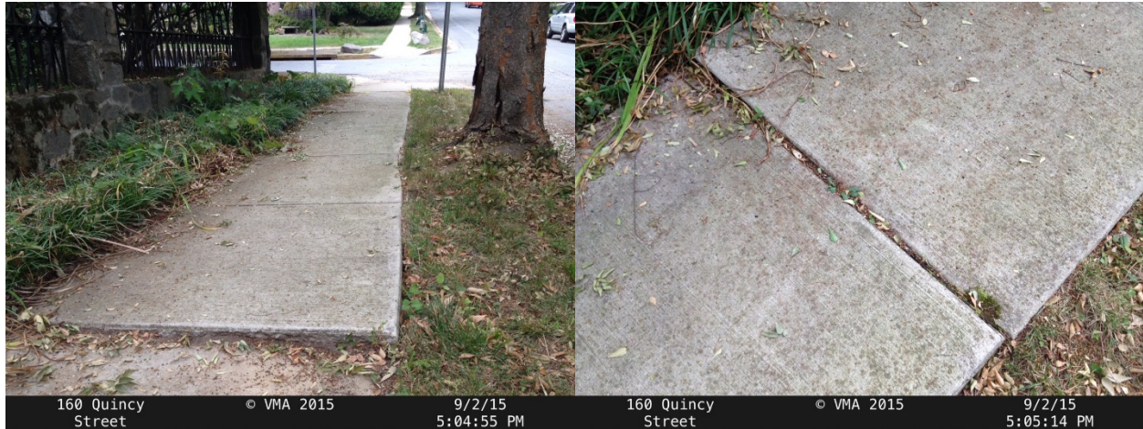
Sidewalk sections pitched by tree roots, grind raised portions.
