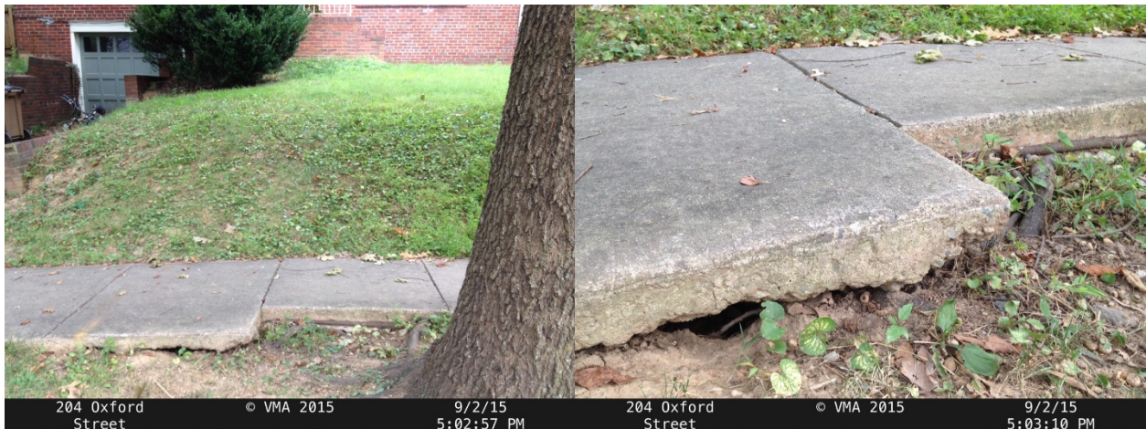
Possible rodent or drainage issues, replace sidewalk sections including new backfill.
