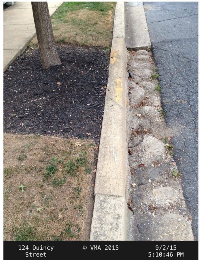
Crumbling, install new currb & gutter section.
