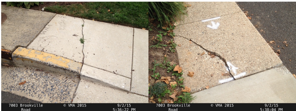
Tripping hazards & graffiti, replace sections.
