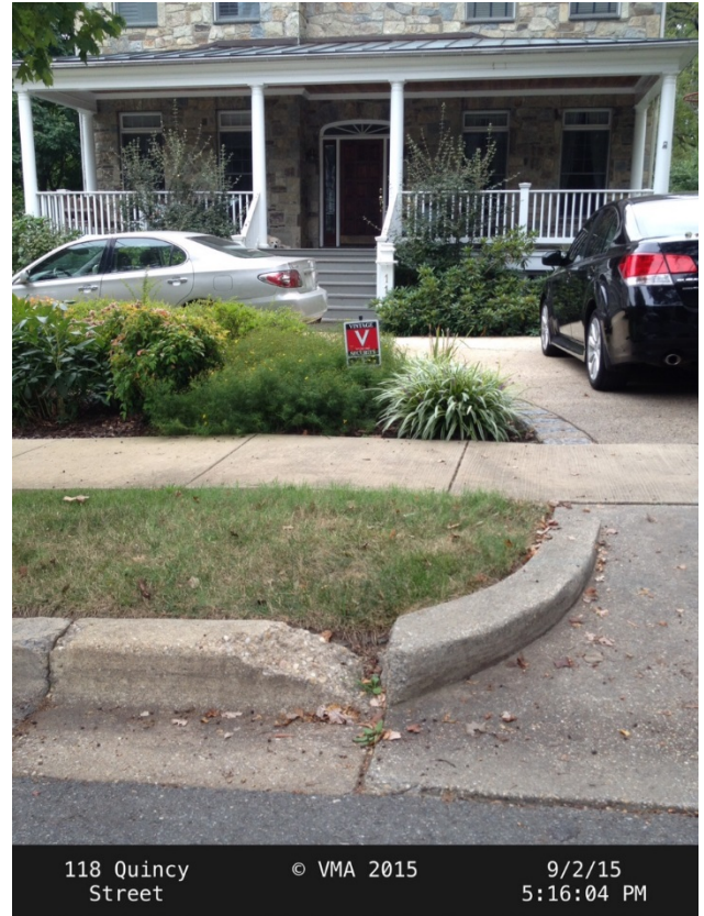
Crumbling, install new currb & gutter section.
