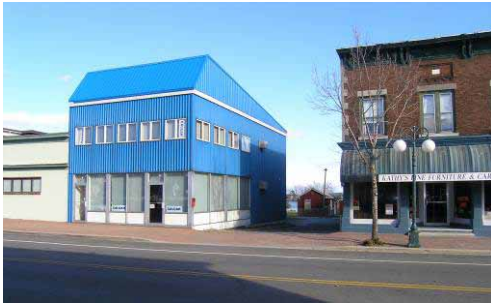
Figure 6 — The current condition of the Calgah Building at 111 Lake Street. The façade is incompatible with the downtown setting.
