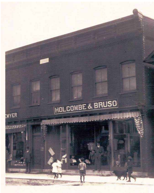
Figure 27 — 93-95 Lake Street historic photo (left), and today (right). The Italianate-style details on the ground floor—windows, entrance, and cornice — have all been covered by modern wood siding, which takes away from the historic charm of the building. It may be possible to expose the original details if this building undergoes renovation. If the façade has degraded beyond restoration, the picture on the left can be a source of inspiration for a more contemporary interpretation of a historic building.
