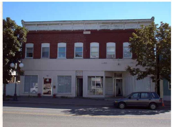
Figure 27 — 93-95 Lake Street historic photo (left), and today (right). The Italianate-style details on the ground floor—windows, entrance, and cornice — have all been covered by modern wood siding, which takes away from the historic charm of the building. It may be possible to expose the original details if this building undergoes renovation. If the façade has degraded beyond restoration, the picture on the left can be a source of inspiration for a more contemporary interpretation of a historic building.
