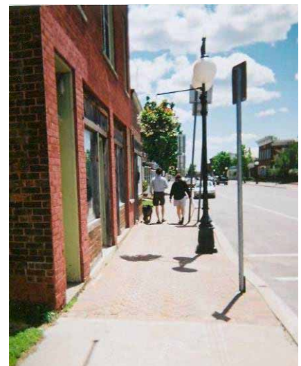
Figure 42 — Existing sidewalk on Lake Street, with concrete pavers at an uneven slope.
