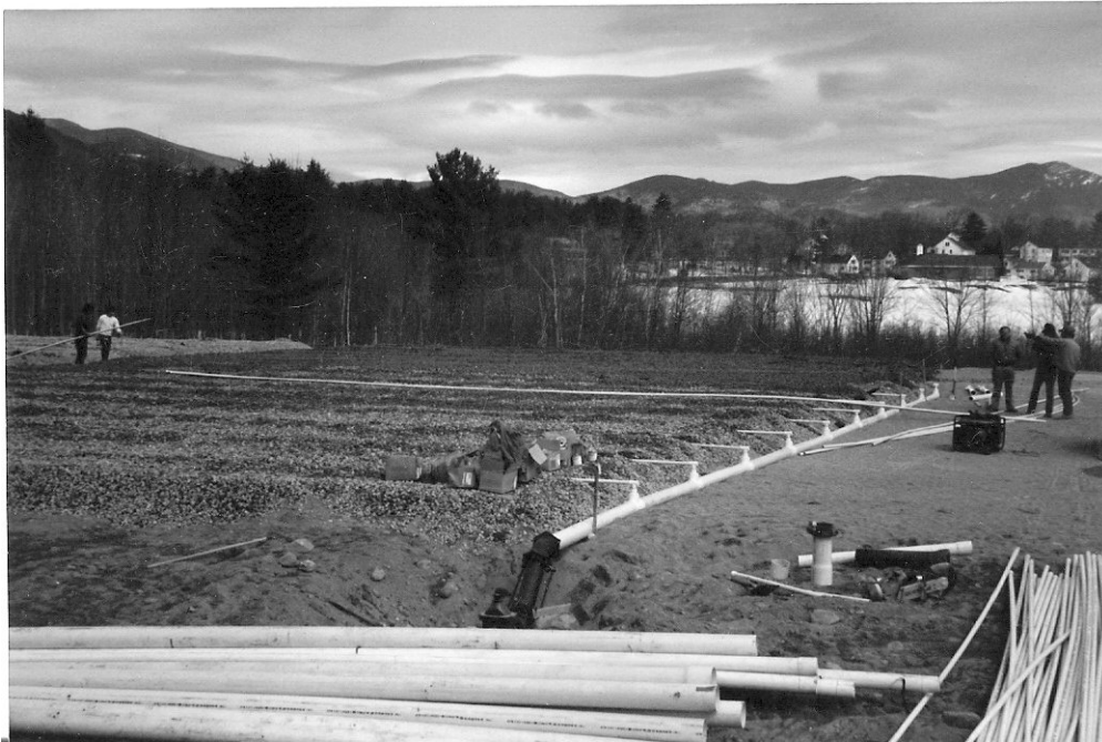
Construction of the Leachfield - 1987
