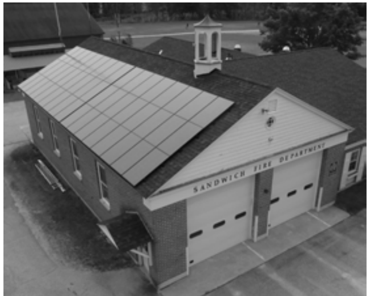
~ Solar Photovoltaic System at the Central Fire Station ~
