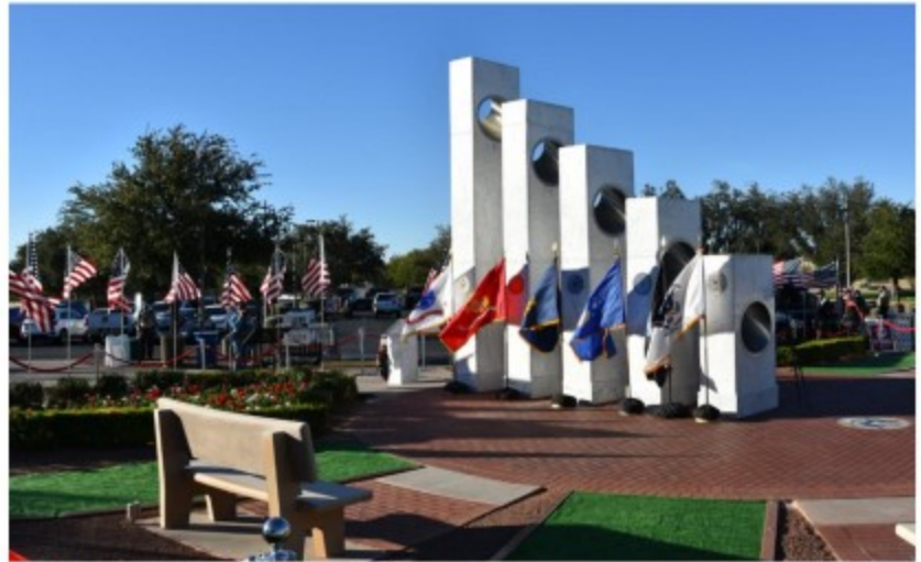
The Anthem Veteran's Memorial is set undergo construction improvements funded by area nonprofit organizations, local business and community residents. An additional 3,000 pavers will be placed.
