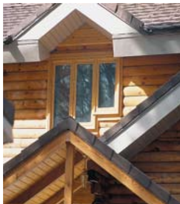
Enclose eaves and soffits.
