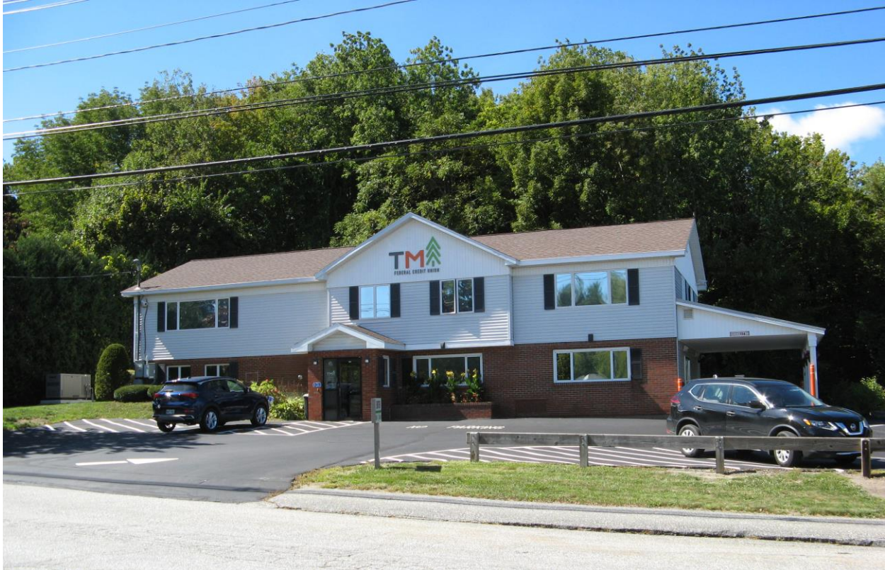
View looking west across Edison Drive at the Trademark Federal Credit Union.
