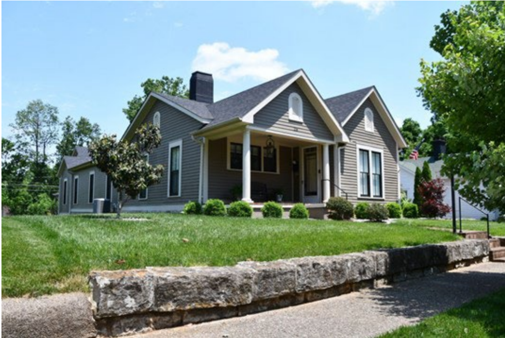
Figure 17. Stone retaining walls can also be found in the district. This wall is along the north side of East Flaget Street. See Guideline 1.6.2 .
