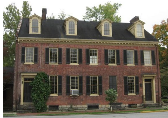
The McLean House at 105 East Stephen Foster Avenue is an outstanding example of Federal period commercial architecture.
