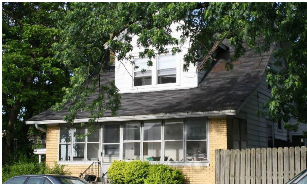
Figure 67. The front porch was enclosed on this bungalow. This type of treatment is not permitted under Guideline 7.1.1.
