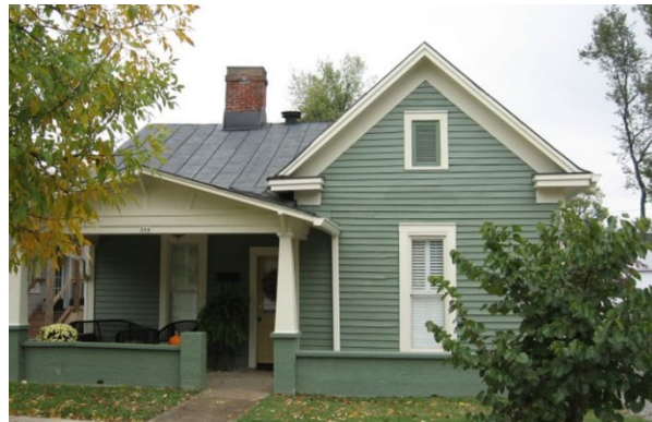
The house at 214 East John Fitch Avenue uses a single story gable-front and wing plan. Its cornice with returns demonstrates Italianate or Greek Revival influences, and the porch, built in the early 20th century, is Craftsman style.
