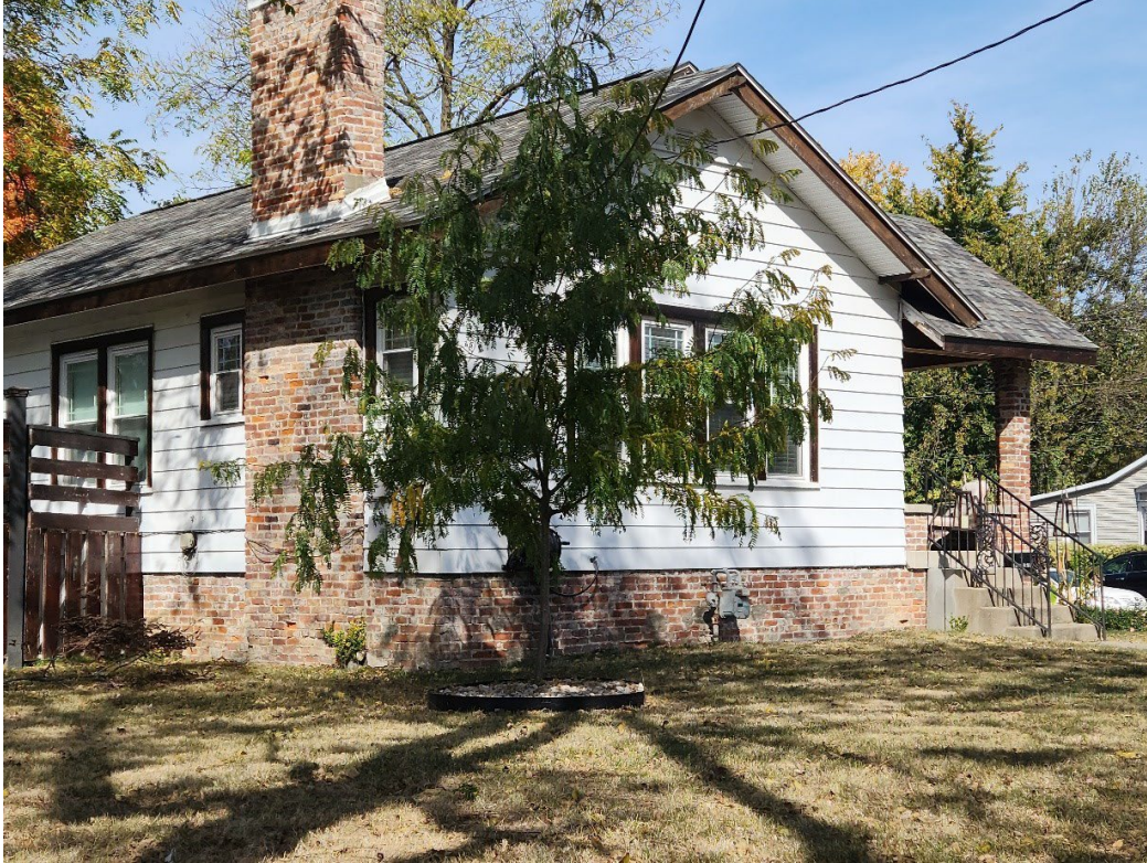
Figure 30. This foundation wall was inappropriately cleaned using an abrasive method and repointed using incorrect materials. See Guidelines 3.2.1 and 3.2.3.
