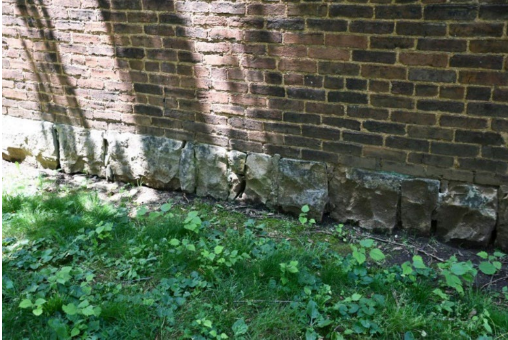
Figure 20. Stone foundation walls are extremely common on 19th century buildings in the Bardstown Historic District. See Guideline 2.1.
