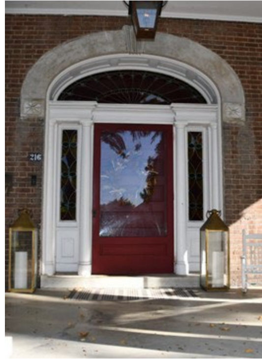
Figure 62. Historic storm door in the Bardstown District. Preservation Guidelines can be found in Guidelines 6.1 and 6.4.1.
