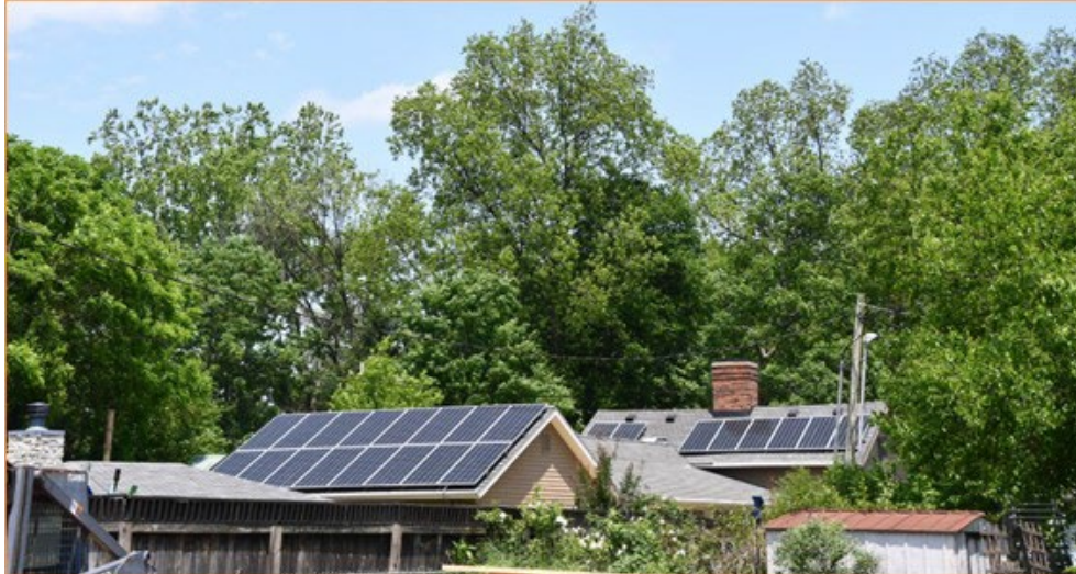
Figure 92. Solar panels can be added to a garage at the rear of a property. See Guideline 11.2.
