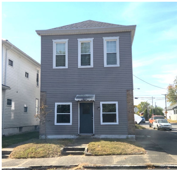
Figure 39. This neighborhood storefront was obscured and (mostly) covered with vinyl siding to convert the first floor to residential space. Note the original brick columns that were left uncovered. This treatment is not in compliance with Guideline 4.1.8 as well as most of Guideline 4.1. See Guidelines 4.1. and 4.2 for information on how to restore this storefront to its former design.
