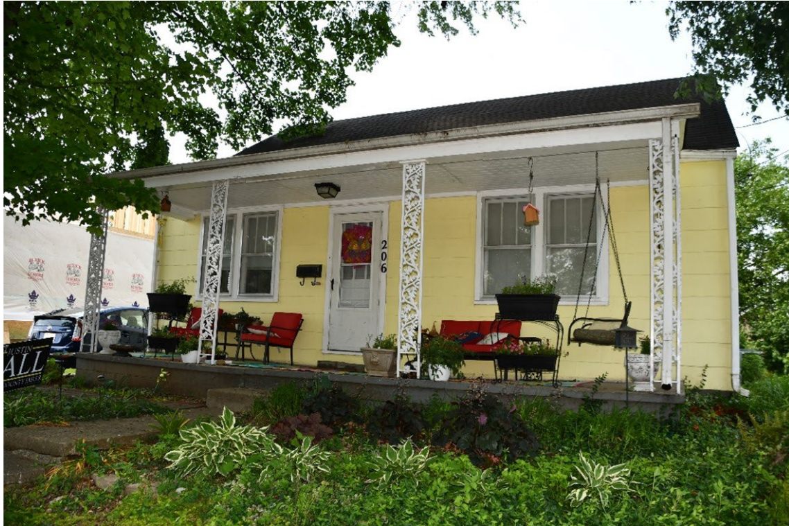
Figure 69. The porch columns on this Bardstown house were replaced by decorative aluminum supports in the mid-to-late 20th century. The original porch likely had wood supports. If restoration is desired, the owner could find similar porches in the area to emulate and examine the current porch for forensic evidence of the original historic porch. See Guidelines 7.2.
