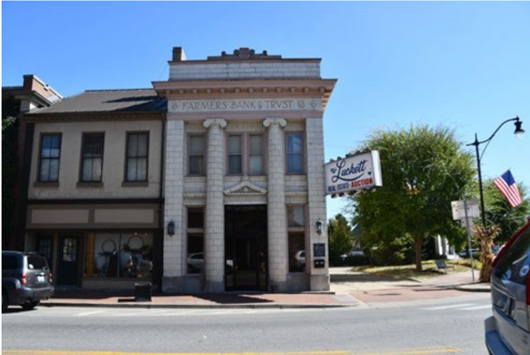
Figure 32. This ceramic veneer building has a decorative cornice line with block modillions, Neoclassical style columns, and a pedimented entryway. For details on their treatment, see Guideline 3.5.
