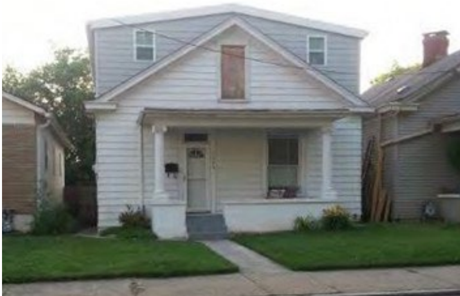
Figure 77. New dormer windows shall not be street-visible and shall not alter the primary façade's historic roof form significantly, like this one does. See Guidelines 8.4.2. In addition, the historic window was covered on the upper story, which is also not permitted under Guidelines 5.5.
