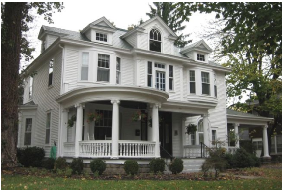
This early Colonial Revival house at 502 North Third Street is an example of the Free Classic style. It demonstrates Federal and Georgian influences in its pedimented dormers, arched windows, transom-and-sidelights opening surround, and Ionic capitals. The asymmetry created by its porches was influenced by the Queen Anne style.
