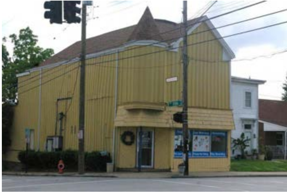
Figure 38. This historic commercial building has been covered with a variety of modern materials, such as an aluminum slipcover and wood shingles. Regardless, the building's 19th commercial form remains intact and the historic building materials are likely intact under the non-compatible modern treatments. See Guideline 4.2 for appropriate treatments to restore this building.
