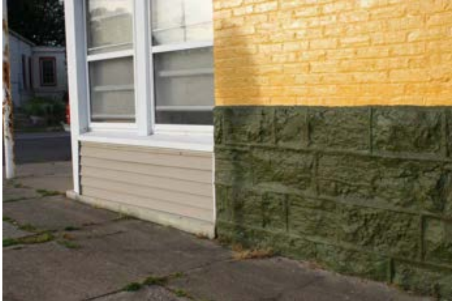
Figure 21. This historic foundation wall has been covered with vinyl (left) and unpainted stone walls have been painted an uncomplimentary color (right). See Guidelines 2.2.1 and 2.3.
