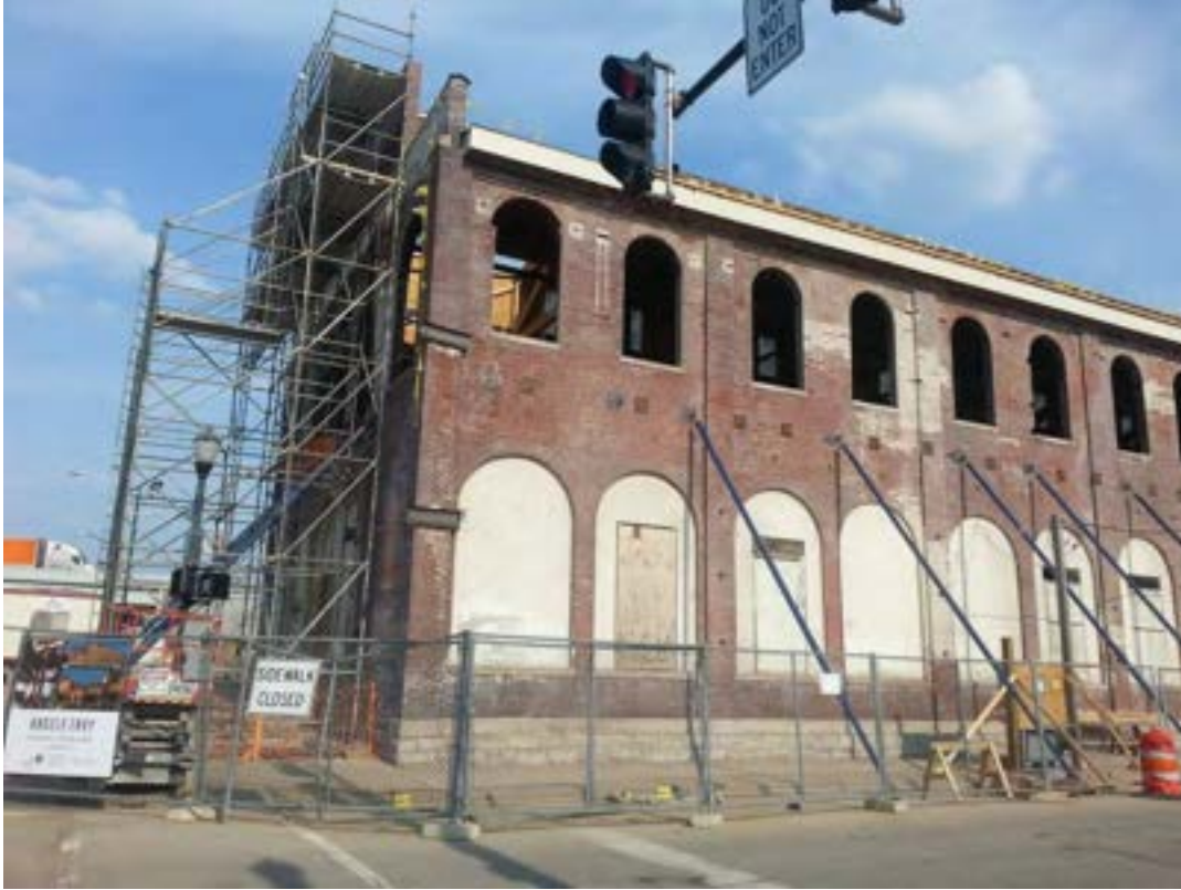
Figure 107. This historic building also experienced demolition by neglect and was gutted in order for the building walls to be preserved. This is only a permitted treatment when the interior has suffered very significant deterioration.
