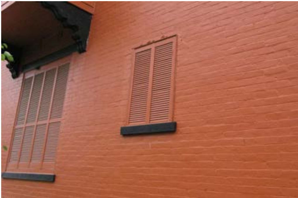
Figure 51. These windows were no longer useful with the new interior program and were covered with shutters so they can be restored when the interior programming needs change. See Guideline 5.5.3.
