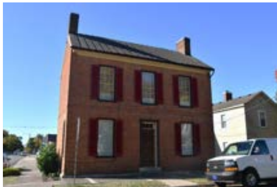
Figure 1. The Horine House (circa 1800) at 201 West Flaget was rehabilitated using guidance from the historic preservation guidelines. The windows and doors were repaired and the standing seam metal roof was stripped and recoated.
