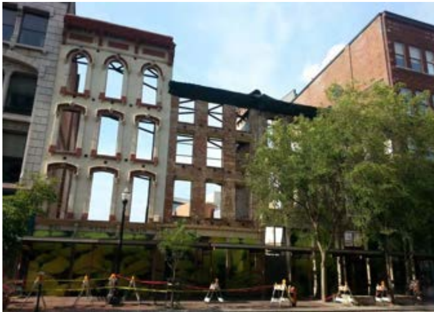
Figure 106. These historic buildings suffered from demolition by neglect. The interiors collapsed and were gutted. The façade and side walls are being preserved so that a new interior program can take place within the historic walls. See Guideline 14.1.6 for information on using historic building walls in new construction.
