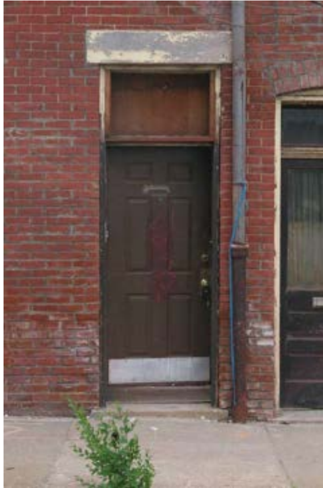
Figure 60. This doorway transom has been covered and the historic door removed and replaced with an inappropriate modern door. An original door can be seen to the right in this photo, which could be used in rehabilitation efforts. These treatments are not permitted under Guidelines 4.1.2, 5.5.2, and 6.2.4 .
