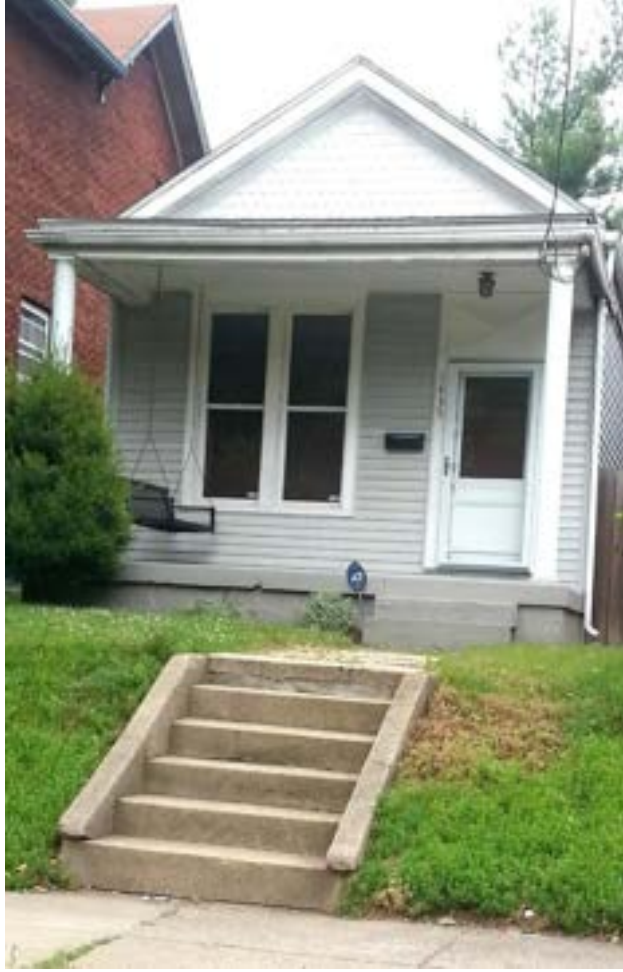
Figure 49. The transom window above the door on this house was covered. This treatment is not permitted under 5.5.2 and 4.1.2.
