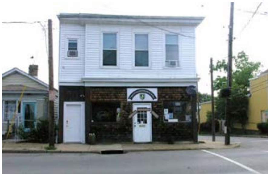
Figure 41. This storefront façade was covered with shake, removing the original display window glass, and the entrance was reduced and replaced. Doors were replaced with modern doors. This treatment is not in compliance with Guidelines 4.2.3 and 4.2.5 as well as most of Guideline 4.1.
