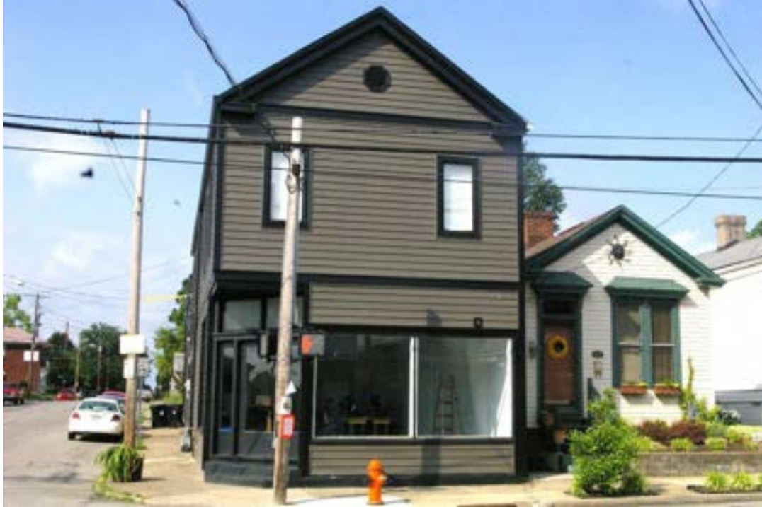
Figure 48. The upper story 2/2 wood windows were reduced in size and replaced by a fixed pane window with a single light. This treatment is not permitted under 5.3.2.
