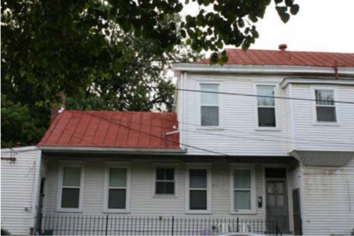
Figure 75. The gutter system is draining directly on the historic standing seam roof. This treatment is prohibited. See Guideline 8.2.5.
