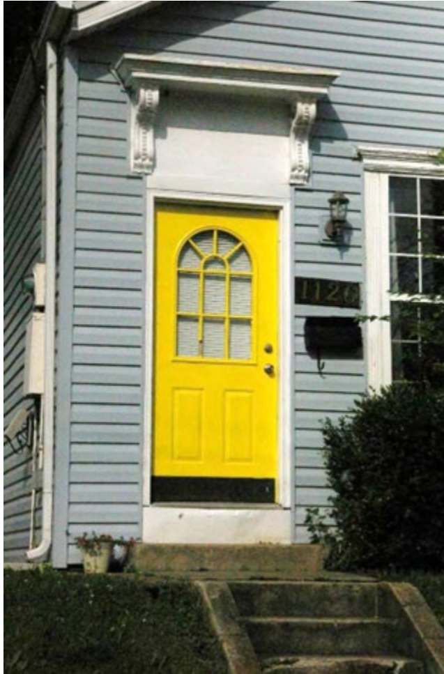
Figure 59 This replacement door is not compatible with the associated historic building. Installing this type of modern metal-clad door on a historic building (and enclosing the transom window) is not permitted under Guideline 6.2.4 and 4.1.2.
