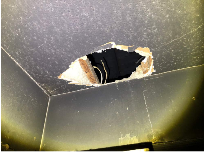
Exposed Electrical Wires
