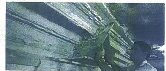
The missing plaster cornice was restored as part of an overall project to return a residence to its original appearance. The traditional method of producing a cornice is unchanged today. Photo: Old-House Journal.
