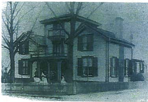
This ca. 1900 photograph (left) would be invaluable to guide restoration of the deteriorated house (right) to its documented earlier appearance, complete with decorative trim, shutters, polychromed exterior, and fencing. Photos: Courtesy, North Carolina Department of Archives and History.
