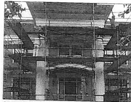
Ongoing work at this house focuses on the maintenance and repair of exterior wood features from the restoration period. After scraping and sanding, the wood was painted in colors documented to the Restoration period. Photo: ©Mary Russell, 1992.
