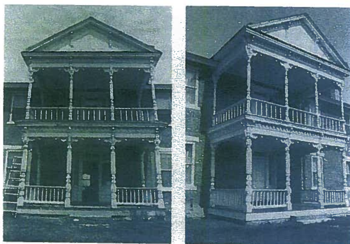
In Rehabilitation, deteriorated features should be repaired, whenever possible, and replaced when the severity of the damage makes it necessary. Here, a two-story porch is seen prior to treatment (left). The floor boards are rotted out and the columns are in a state of collapse, supported only by crude, temporary shafis. Other components are in varying stages of decay. Appropriate work on the historic porch (right) included repairs to the porch rails; and total replacement of the extensively deteriorated columns and floor boards. Some dismantling of the porch was necessary.
