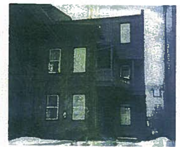
If a rear elevation of a historic building is distinctive and highly visible in the neighborhood, altering it may not meet the Standards. (a and b) This 3-story brick rowhouse featured a second story gallery and brick kitchen wing characteristic of other residences in the district which backed onto a connecting roadway. (c) In the rehabilitation, the wing and gallery were demolished and a large addition constructed that severely impacted the building's historic form and character.
