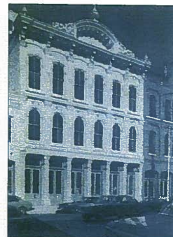
In the treatment, Rehabilitation, one option for replacing missing historic features is to use pictorial documentation and/or physical evidence to re-create the historic feature. (a) In this example, the ornamental cornice of an 1866 limestone building was missing, and the ground level storefront had been extensively altered. (b) and (c) Based on the availability of photographic and other documentation, the owners were able to accurately restore the cornice and storefront to their historic configuration. A substitute material, fiberglass, was used to fabricate the missing pressed metal cornice, an acceptable alternative in this project. All work met the Standards.
