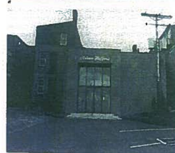
If a rear elevation of a historic building is distinctive and highly visible in the neighborhood, altering it may not meet the Standards. (a and b) This 3-story brick rowhouse featured a second story gallery and brick kitchen wing characteristic of other residences in the district which backed onto a connecting roadway. (c) In the rehabilitation, the wing and gallery were demolished and a large addition constructed that severely impacted the building's historic form and character.
