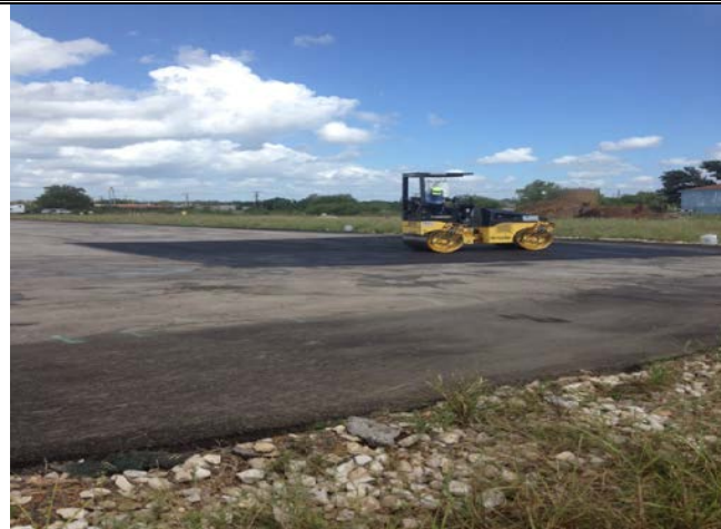
Photo 35: Facing northwest. View of asphalt being compacted on northeast corner of the HMA cover.
