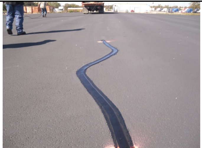
Photo 52: View of crack sealant applied to existing crack after settling occurred.
