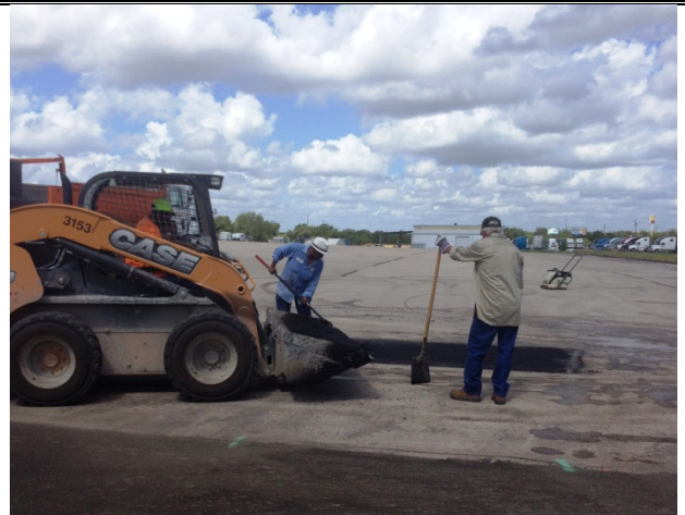
Photo 30: Facing west. View of contractors patching milled cracks.
