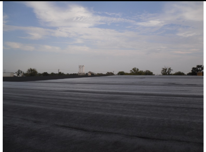
Photo 44: Facing northwest. View of seal coat application on the HMA cover.
