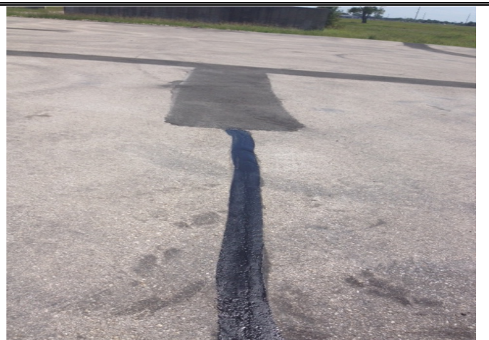
Photo 42: Facing east at a sealed crack.
