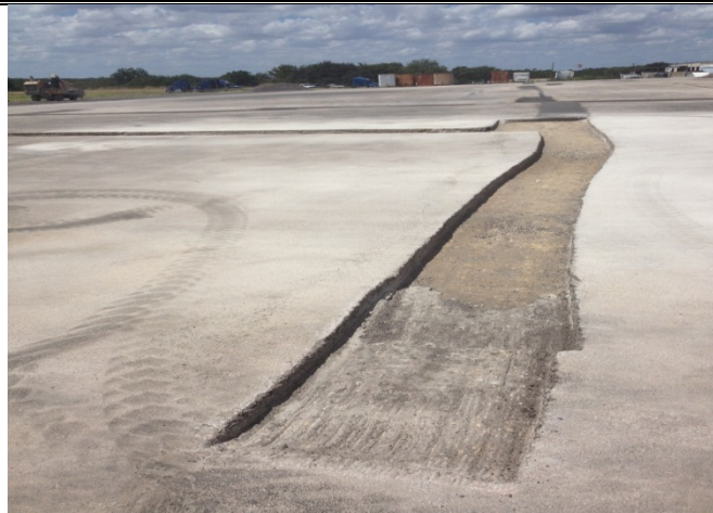
Photo 29: Facing west at milled and compacted crack areas located on the HMA cover.
