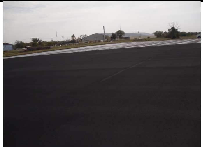
Photo 46: Facing northeast. View of final seal coat curing and drying.
