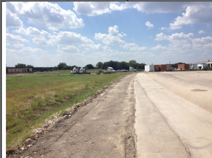
Photo 21: Facing west at the southern side of the milled and compacted apron.
