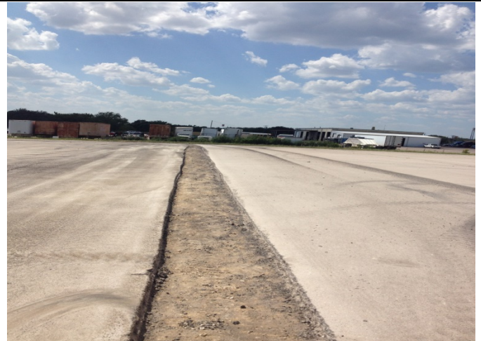
Photo 28: Facing west at milled and compacted crack areas located on the HMA cover.
