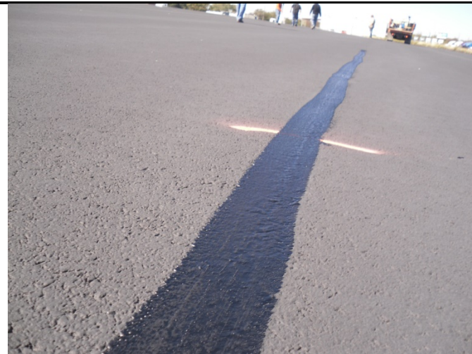
Photo 51: View of crack sealant applied to existing crack after settling occurred.
