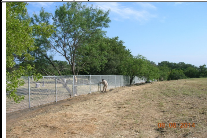
Photo 17: Facing northwest as contractor secures chain-link fence to fence posts.
