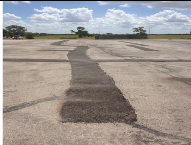
Photo 31: Facing east. View of milled areas filled with asphalt during patching and overlay activities.
