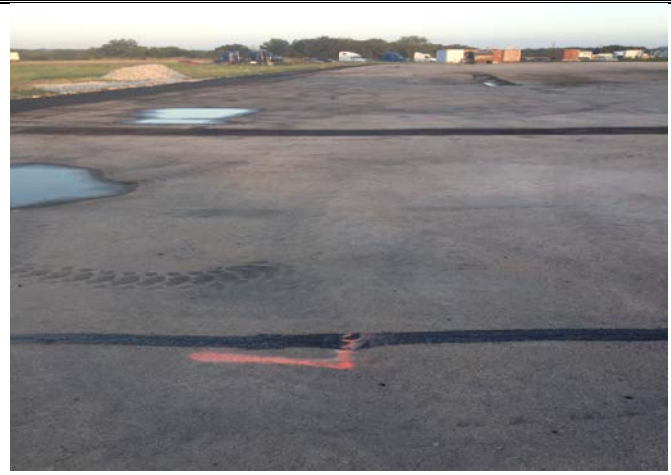
Photo 36: Facing west at depression on the southern side of the HMA cover.
