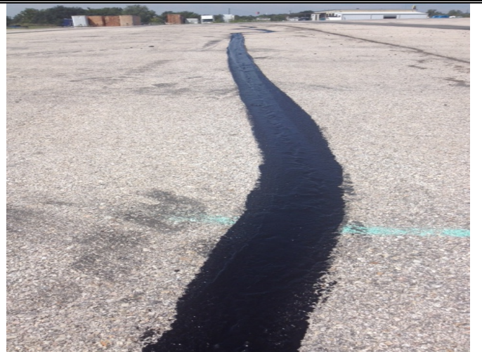
Photo 40: Facing west at a sealed crack.
