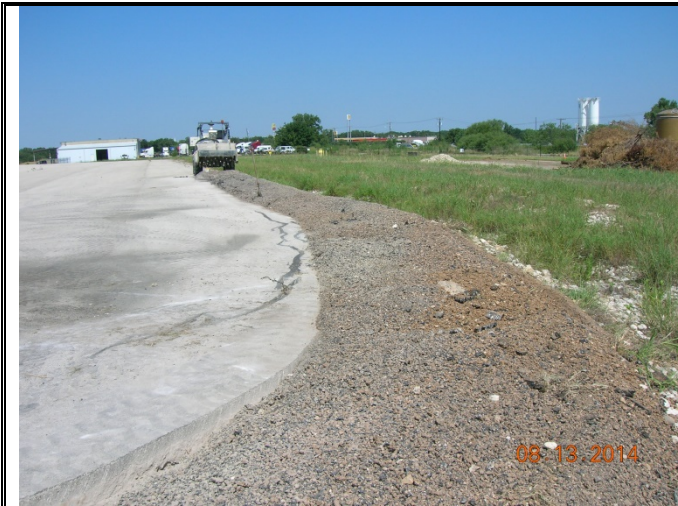
Photo 19: Facing northwest on north-side as contractor mills the 7-foot apron surrounding the HMA cover.
