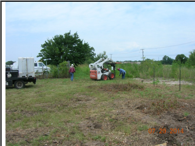
Photo 13: Facing northwest at contractors drilling hole for barbed wire fence on south property.
