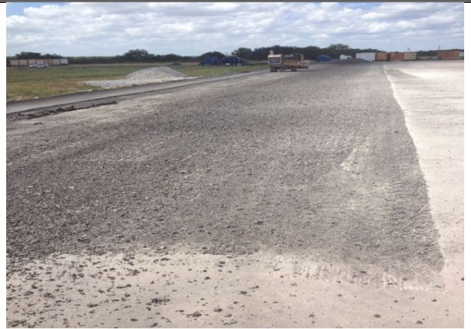
Photo 38: Facing southwest at southern depression being milled.
