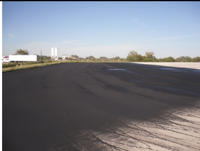
Photo 43: Facing west. View of seal coat application on the HMA cover.
