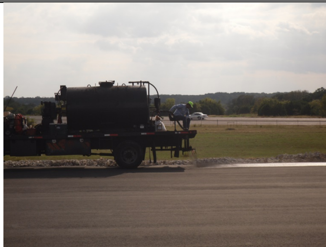
Photo 45: Facing south. View of crew applying final seal coat on the HMA cover.
