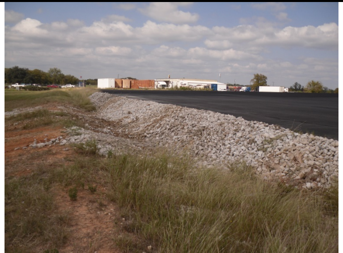
Photo 50: Facing west. View of constructed and re-enforced rip-rap located on the southern side of the HMA cover.
