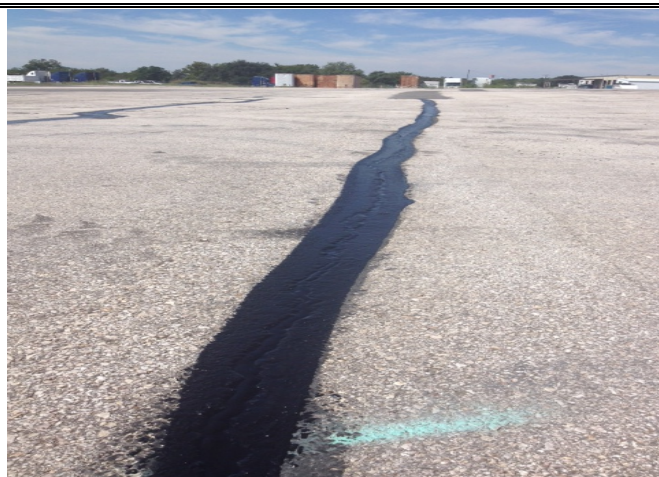
Photo 41: Facing west at a sealed crack
