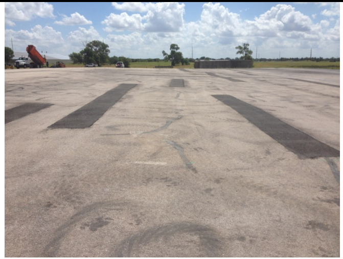
Photo 32: Facing east. View of milled areas filled with asphalt during patching and overlay activities.
