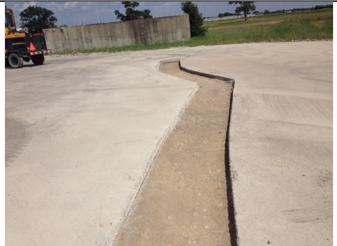
Photo 26: Facing east at milled and swept crack areas located on the HMA cover.
