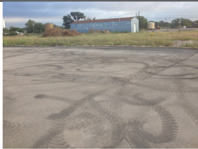
Photo 34: Facing northwest looking at milled depression on northeast corner of the HMA cover.
