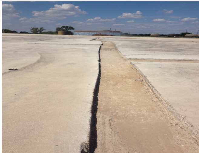
Photo 25: Facing north at milled and swept crack areas located on the HMA cover.
