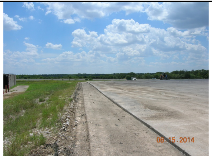
Photo 20: Facing south at the eastern side of the milled and compacted apron.
