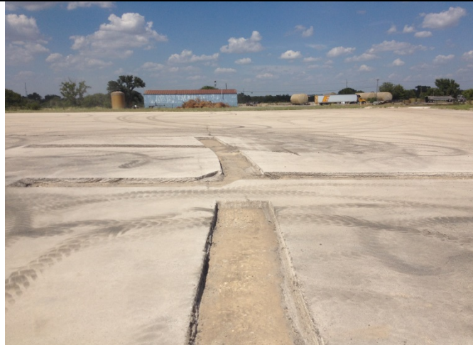
Photo 27: Facing north at milled and compacted crack areas located on the HMA cover.
