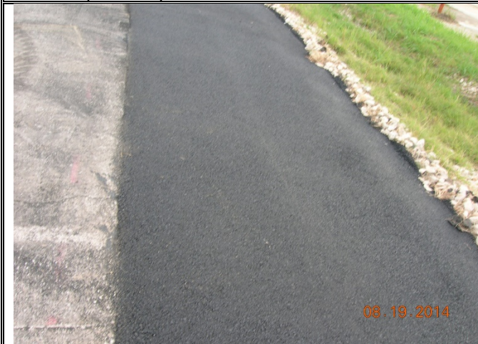
Photo 23: Close-up view of newly laid and compacted asphalt.
