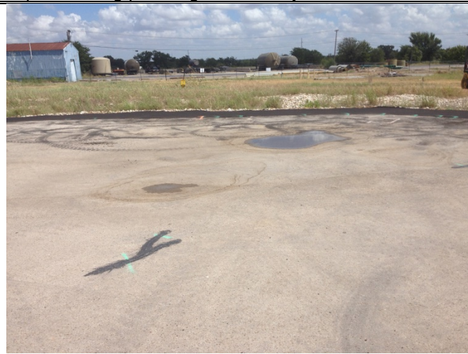
Photo 33: Facing northeast. View of depression on northeast corner of the HMA cover.
