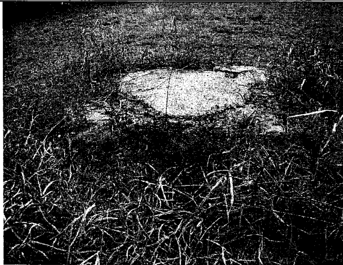
Photo #7 Date: November 23, 2010 Description: Plugged manhole on east side of the North Property
