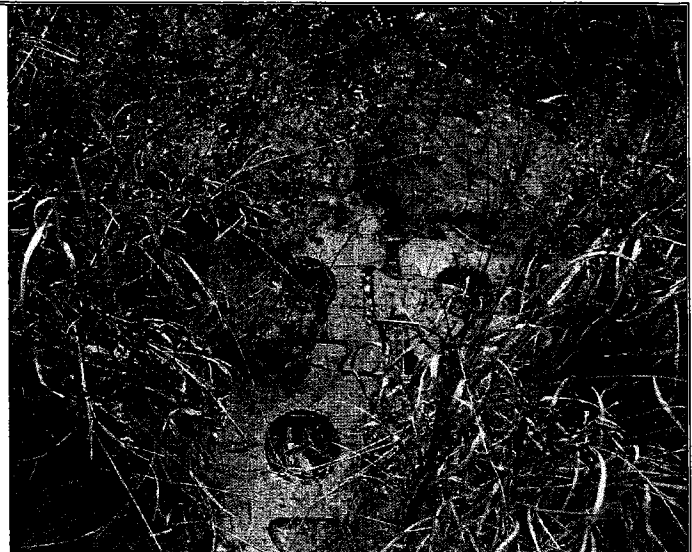
Photo #18 Date: November 23, 2010 Description: Articulated blocks along Leon River embankment.
