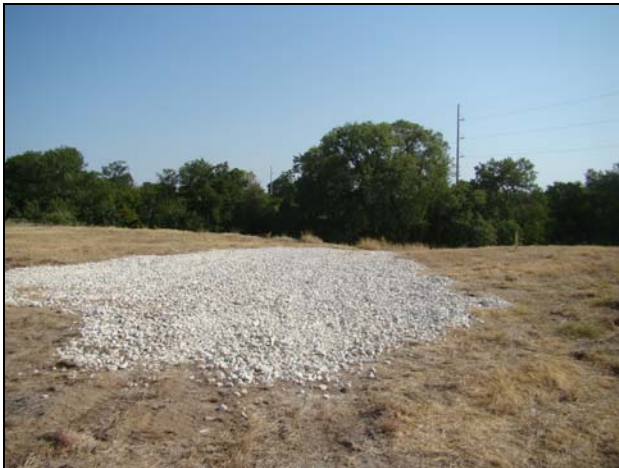
Photo #27 Date: August 3, 2011 Description: Looking North at North Property Coarse Gravel Installation for Runoff and Erosion Control.
