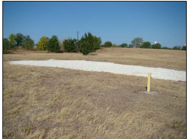
Photo #28 Date: August 3, 2011 Description: Looking Southwest at North Property Coarse Gravel Installation for Runoff and Erosion Control.
