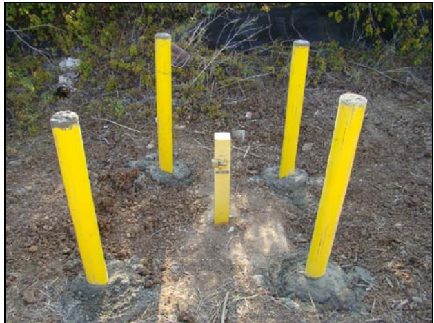
Photo #16 Date: August 3, 2011 Description: Looking West at MW-29-90 on the Central Property with Bollards Installed and Vegetation Removed.
