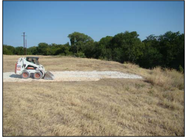
Photo #26 Date: August 3, 2011 Description: Looking Northwest at North Property Coarse Gravel Installation for Runoff and Erosion Control.
