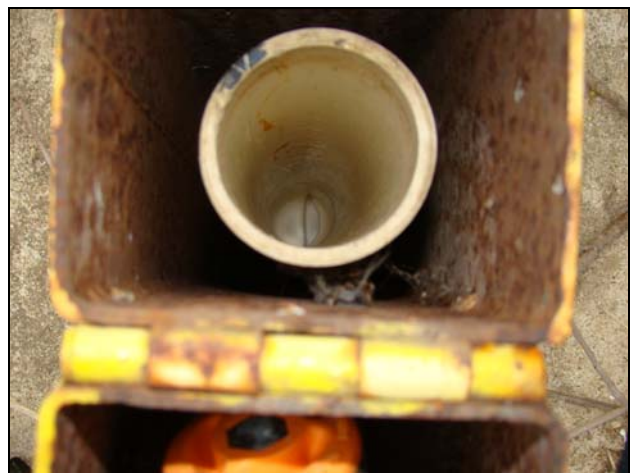
Photo #16 Date: May 2, 2011 Description: Looking at Obstruction Located Inside Well Casing at MW-36-90 on the North Property.
