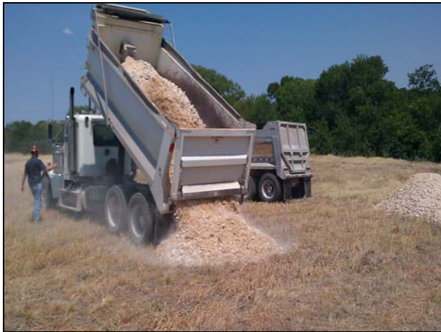
Photo #23 Date: August 3, 2011 Description: Looking Northwest at North Property Coarse Gravel Installation for Runoff and Erosion Control.
