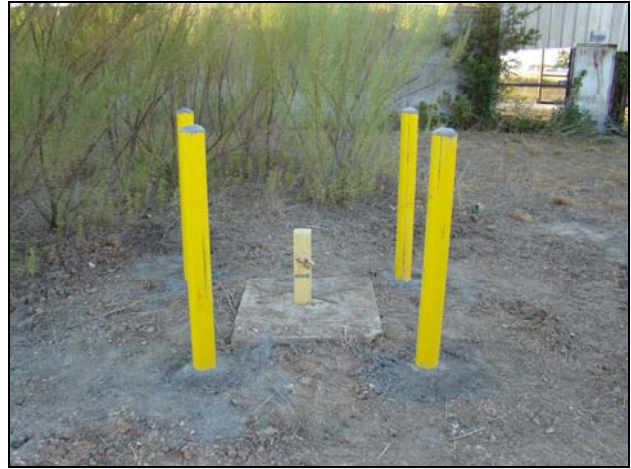
Photo #18 Date: August 3, 2011 Description: Looking West at MW-30-90 on the Central Property with Bollards Installed and Vegetation Removed.
