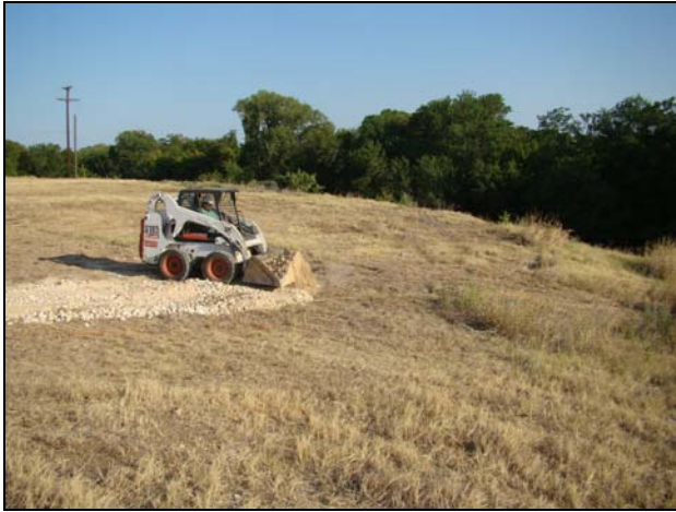
Photo #25 Date: August 3, 2011 Description: Looking Northwest at North Property Coarse Gravel Installation for Runoff and Erosion Control.
