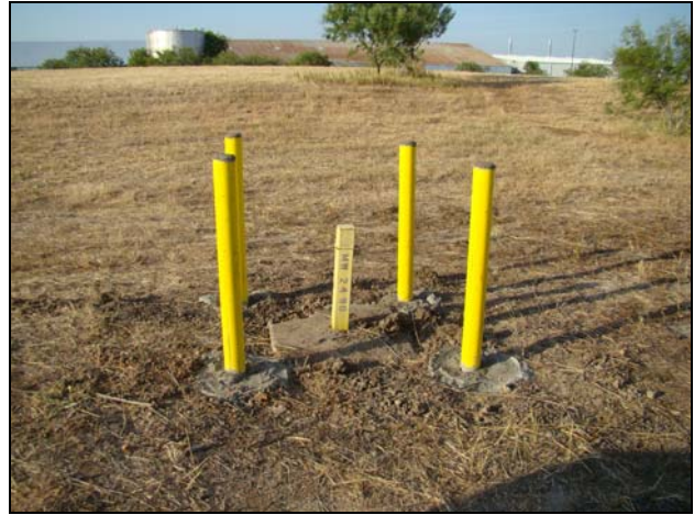
Photo #10 Date: August 3, 2011 Description: Looking North at MW-24-90 on the Central Property with Bollards Installed and Vegetation Removed.
