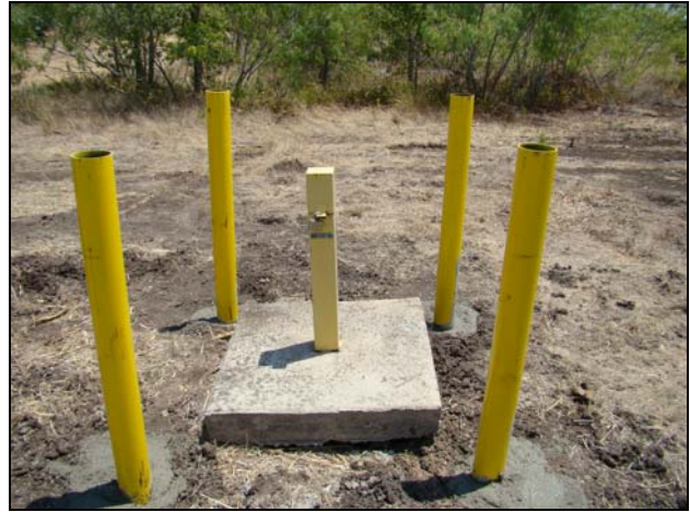
Photo #22 Date: August 3, 2011 Description: Looking Northeast at MW-34-90 on the Central Property with Bollards Installed and Vegetation Removed.
