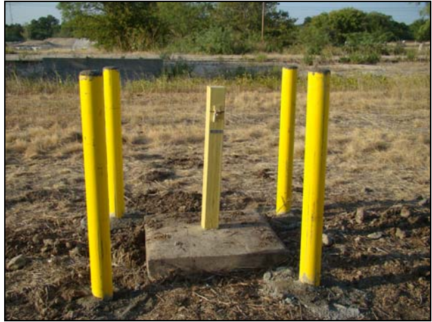
Photo #14 Date: August 3, 2011 Description: Looking North at MW-28-90 on the Central Property with Bollards Installed and Vegetation Removed.
