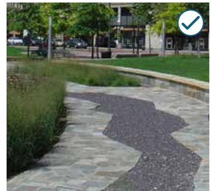
Incorporate Low Impact Development (LID) principles, such as stormwater planters and permeable pavement, to mitigate stormwater impacts.
