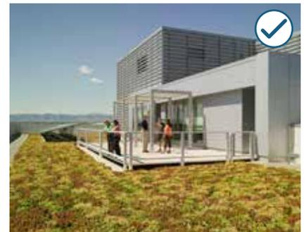
Design building projects to reduce stormwater runoff by including a greenroof.
