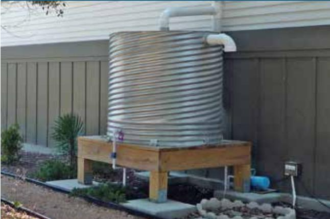
Rain barrels are storage devices that collect rain water for reuse in lawn and garden watering or other uses. They are generally connected to roof gutter systems.
