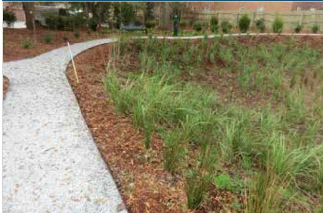
Bioretention systems manage and treat stormwater runoff in a shallow depression filled with a soil bed and planting materials to filter runoff. They help provide greater site utilization and attractive landscape areas while protecting water quality.
