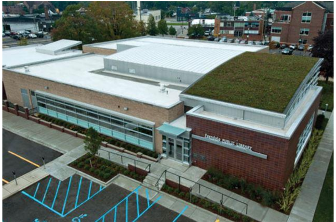
Seedum installed on Ferndale Public Library expansion
