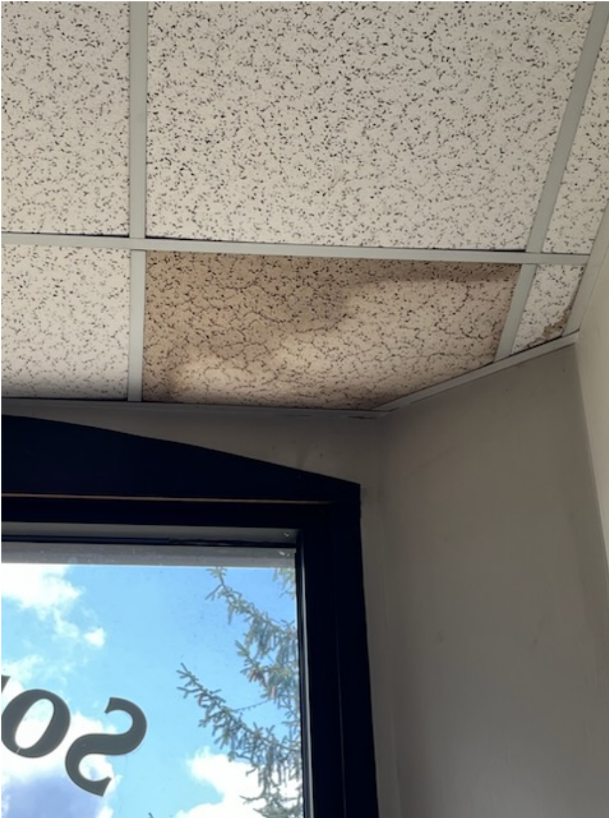
Front Entry Way, has the worst leak, with a bowing ceiling tile.
