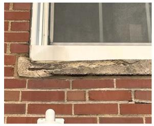
• The water has infiltrated some of the sills and caused it to deteriorate to the point where large chunks of precast have fallen off and the rebar is exposed. Once rebar is exposed, the rusting of the rebar will accelerate causing the rebar to expand which in turn will cause more cracking and deterioration of the precast. This will also allow water to infiltrate the wall system causing damage there too.
