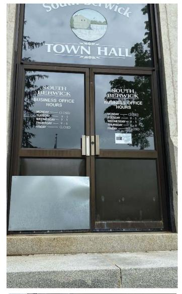
The aluminum storefront front doors are deteriorating, a panel has corroded, and the door should be replaced.
