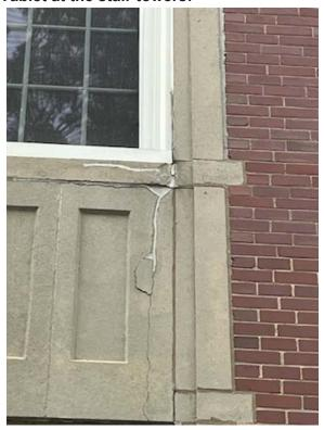
• While pieces have not fallen yet, the large cracks are allowing water into the wall / precast system, and it will continue to crack until it also fails.
