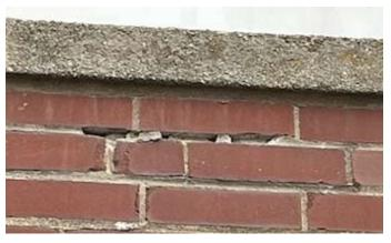
• At places, water has infiltrated the precast concrete and has started to weep through the brick causing the mortar joints to deteriorate. When the precast concrete is stabilized, any places where the mortar is failing will need repointed.
