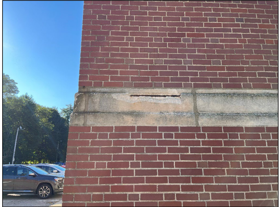
Photograph 1 – Concrete Banding Deterioration
