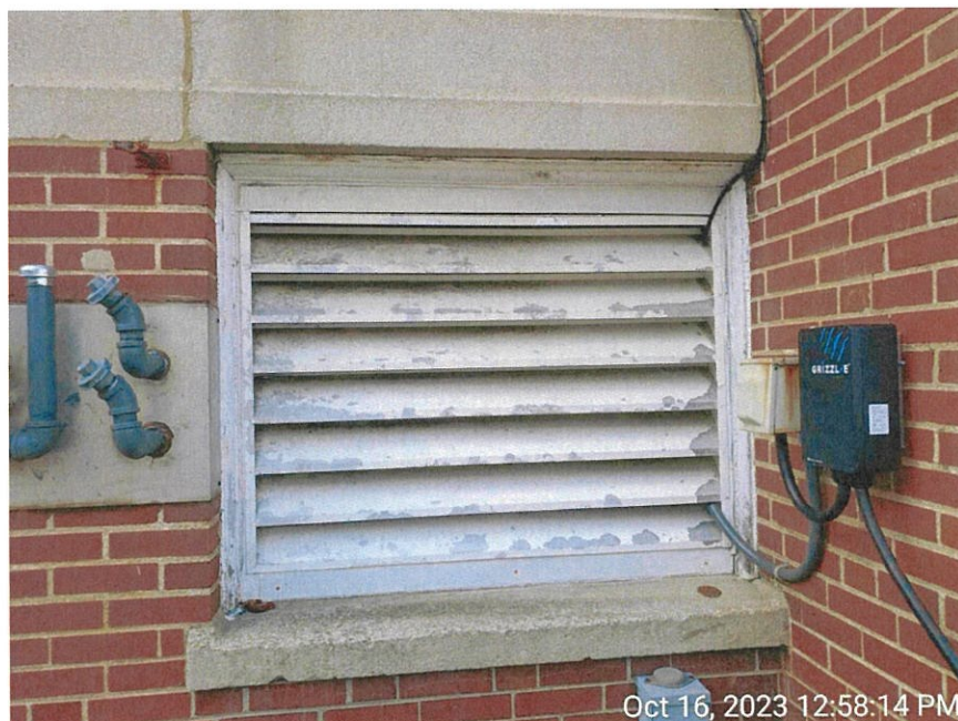
Possible lead-based paint for uncladded wood trim.
