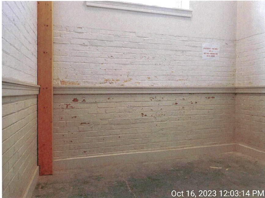
Moisture influences in first floor area causing peeling paint conditions.
