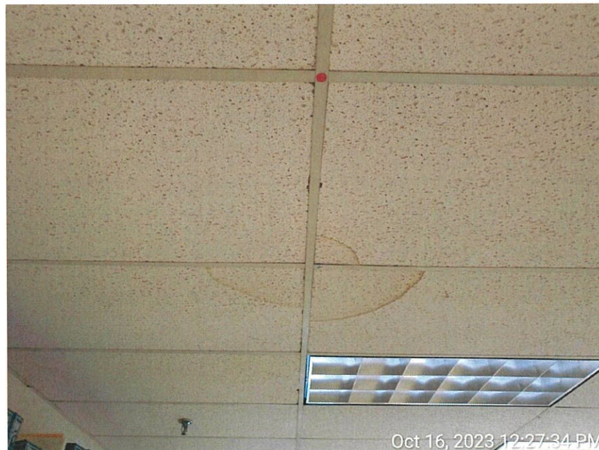
Water-stained ceiling tiles dirty return diffuser and ductwork on second floor in Town Clerk Offices.
