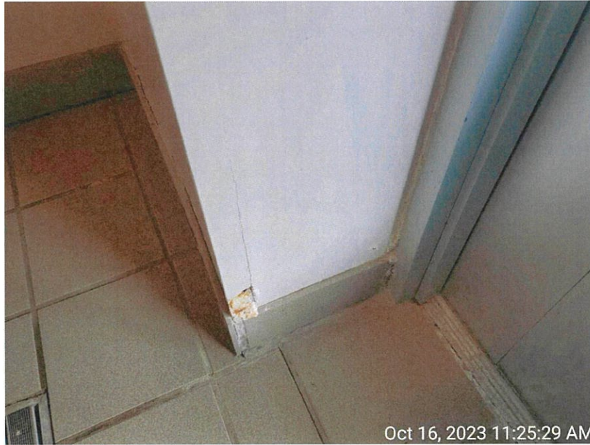
Water damaged lower wall plaster due to improperly sealed door threshold at first floor entry to elevator lobby area.
