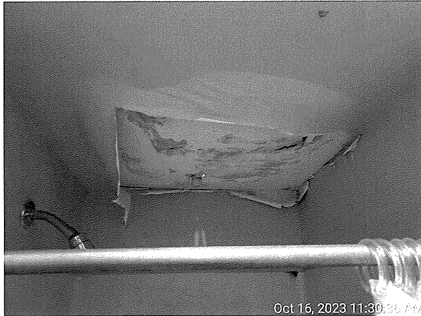
Water damage ceiling in shower unit in first floor former Police locker room.
