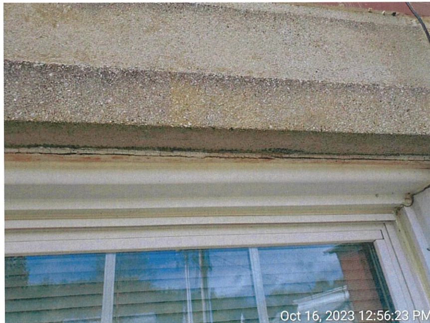
Shrinking/cracking window caulking for header area is rainwater intrusion point.
