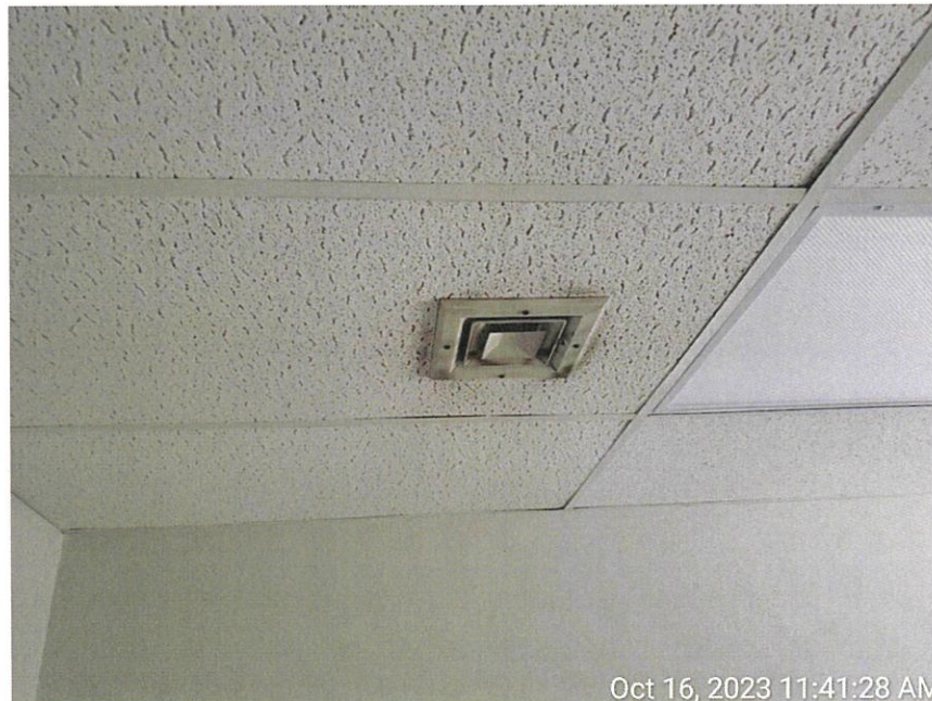
Dirty supply diffuser and ductwork on first floor in former Police Interview Room.
