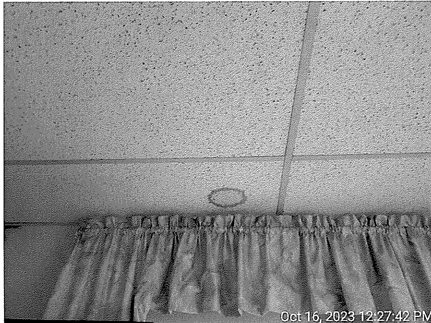
Water-stained ceiling tile on second floor in Town Clerk Offices.
