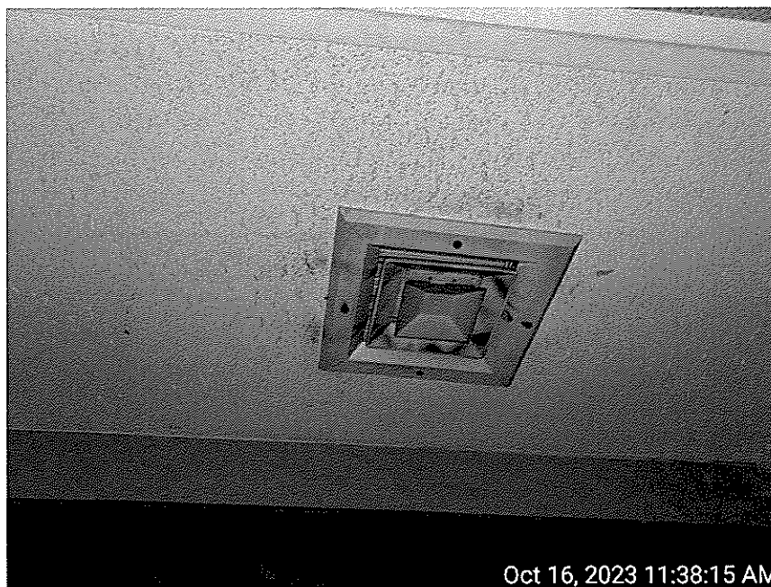
Dirty supply diffuser and ductwork on first floor in Utility Room near former Police Patrol Office.
