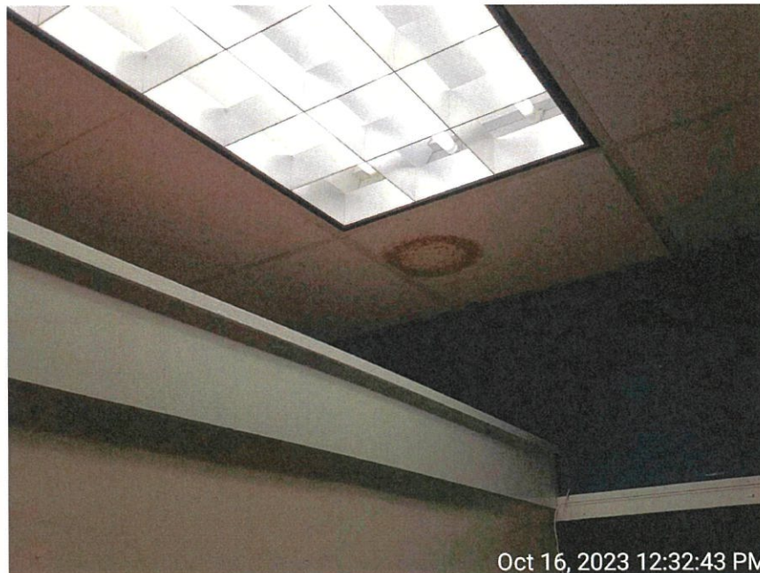
Water-stained ceiling tile on second floor in Codes/Planner Offices.
