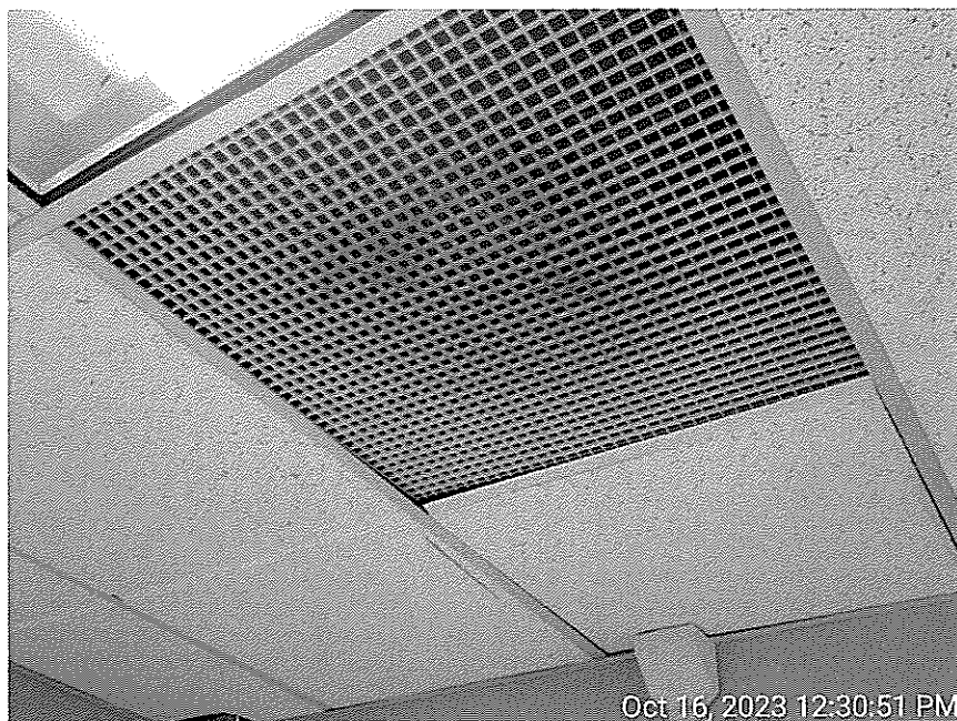
Dirty return diffuser and ductwork on second floor in Assessing Offices.
