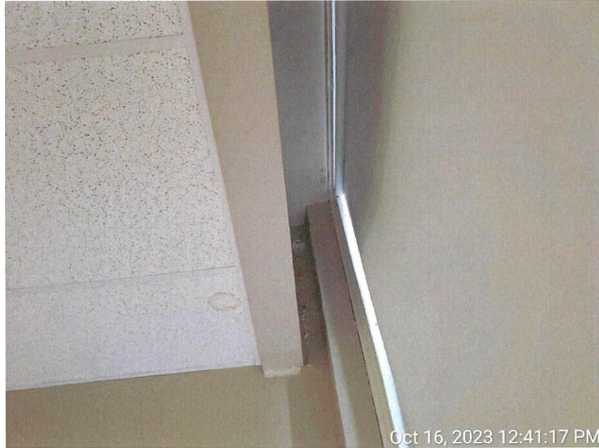
Water intrusion impact for window header on thirld floor In electlon storage room.
