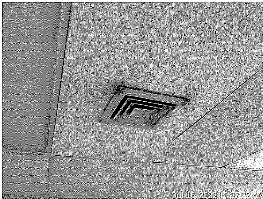
Dirty supply diffuser and ductwork on first floor in former Police Patrol Office.
