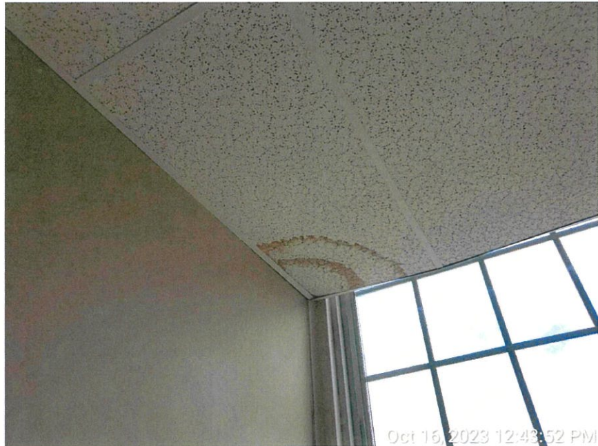
Water damaged ceiling tile on third floor in janitors' storage room.
