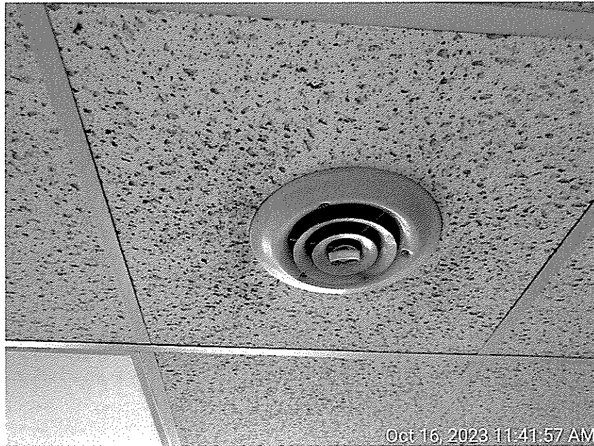
Dirty supply diffuser and ductwork on first floor in former Police Lieutenant & Sergeant Office.
