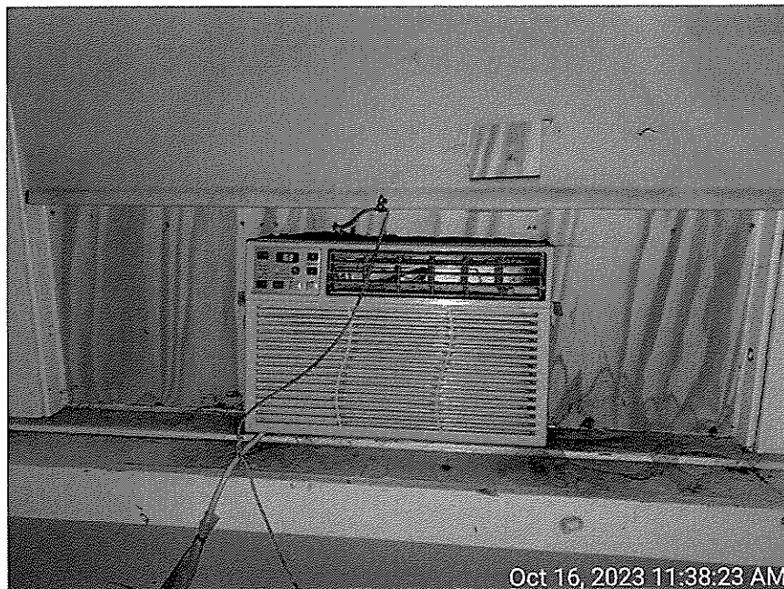
Dirty/mold compromised portable window A/C unit on first floor in Utility Room near former Police Patrol Office.
