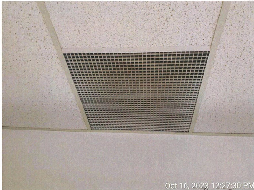
Dirty return diffuser and ductwork on second floor in Town Clerk Offices.
