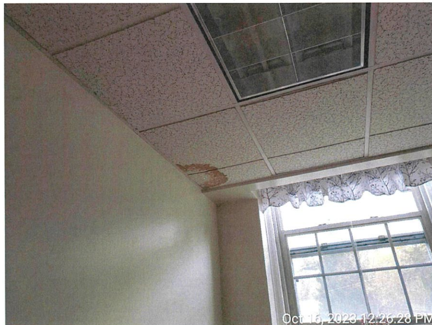
Water damaged ceiling tile on second floor in General Assistance Office.
