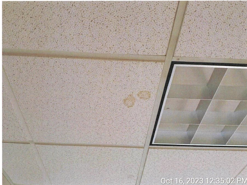
Water-stained ceiling tiles on second floor in Twon Manager Offices.
