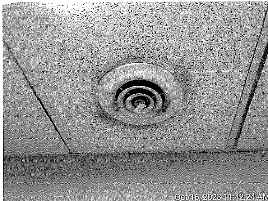
Dirty supply diffuser and ductwork on first floor in former Police Storage Room.
