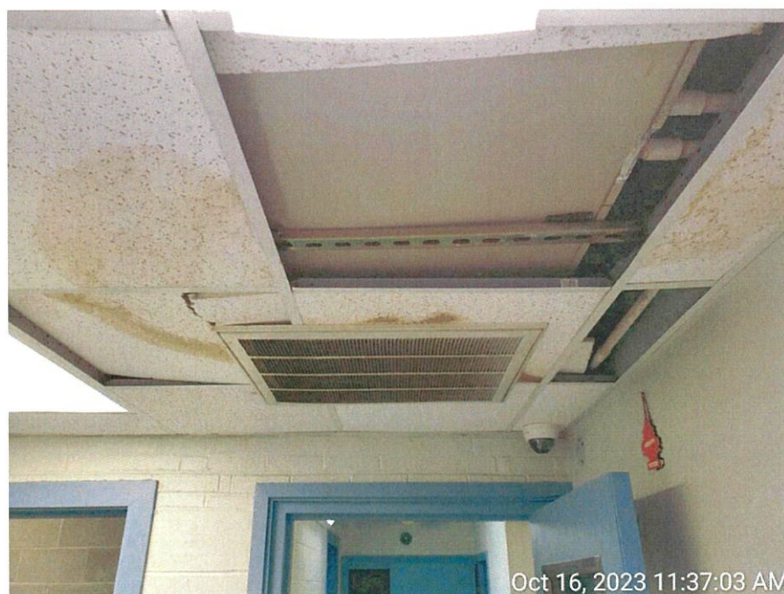
Moisture damaged ceiling tiles due to air handler unit in ceiling on first floor outside former Police Dispatch Office.
