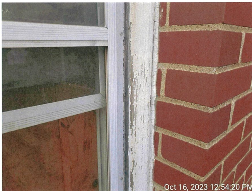
Possible lead-based paint for uncladded window trim.
