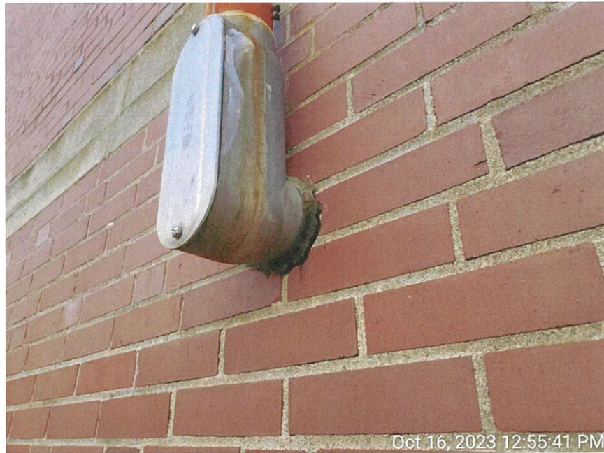
Unsealed perimeter penetrations.
