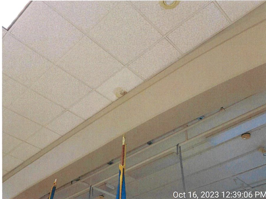
Water-stained ceiling tile on third floor in Auditorium/Stage area. Possible Cladosporium or Stachybotrys mold growth – inaccessible for direct sampling.
