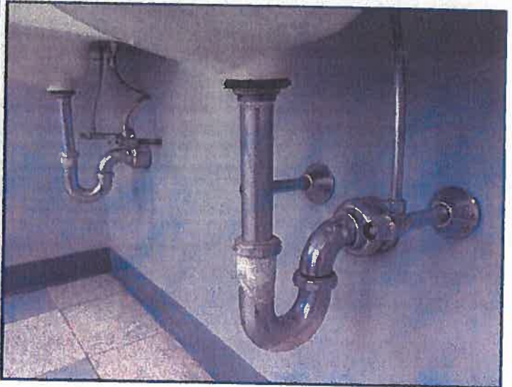
Corrosion of plumbing pillow sinks at third floor men's room.
