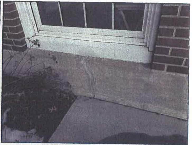
Vertical crack at right side
