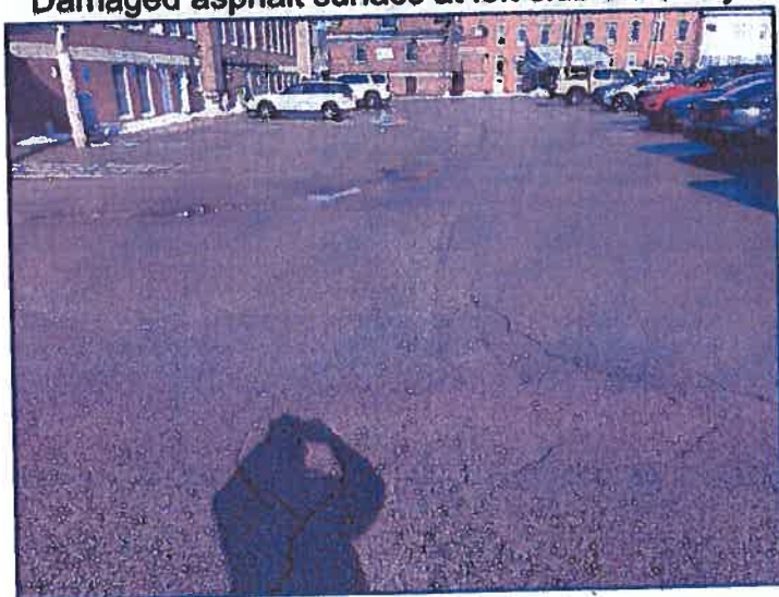
Damaged asphalt surfaces at rear parking
