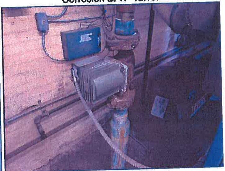
Corrosion at circulator pump.
