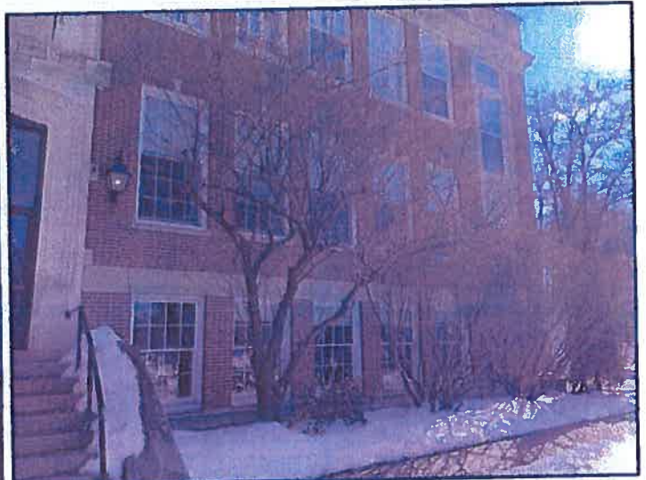
Vegetation in contact with building should be cut back or removed.
