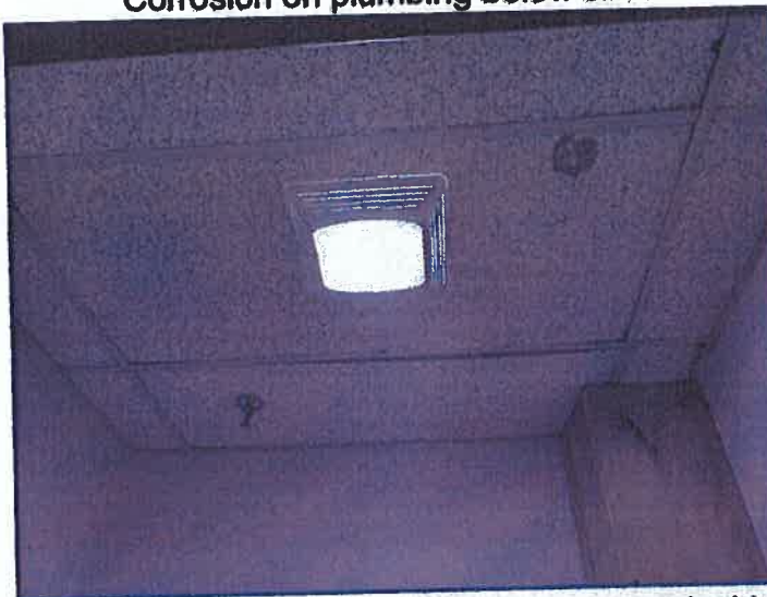
Second floor bathroom vent fans terminate inside building.
