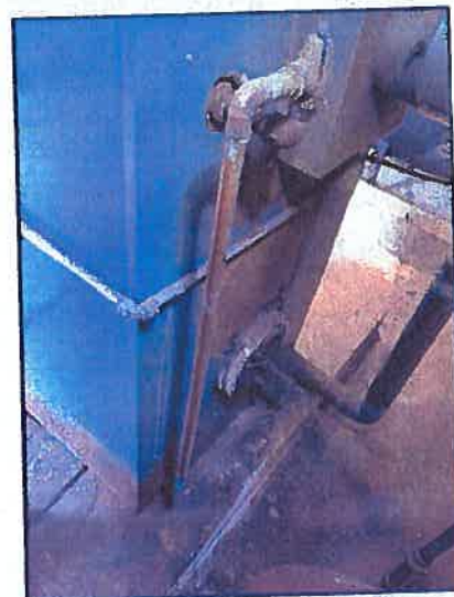
Corrosion at TP valve.
