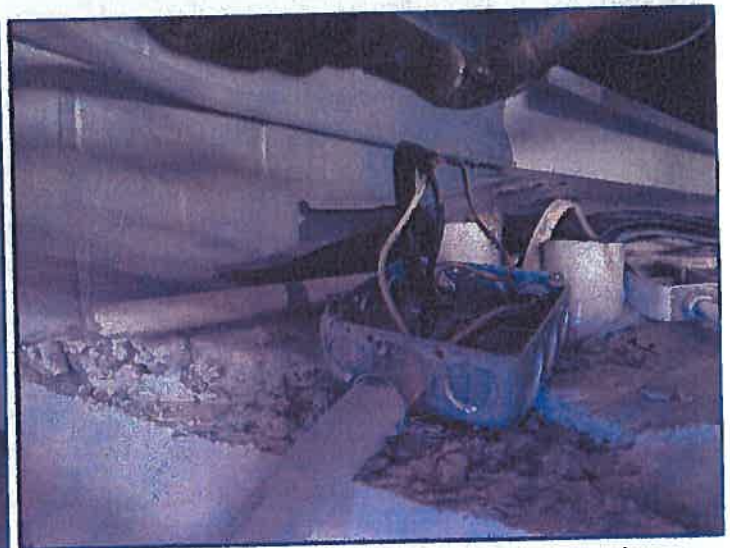
Open junction box at former police station
