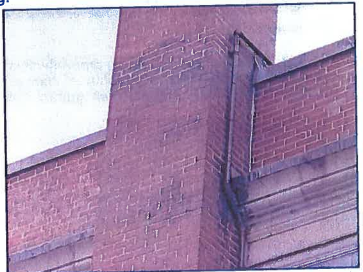
Areas of damage/deterioration to mortar.
