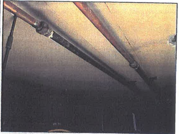
Corrosion on plumbing above drop ceiling at second floor conference room.
