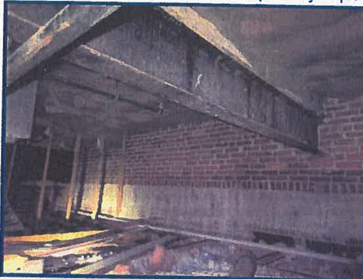
steel beam on masonry wall
