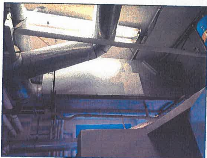
ERV at police station bathroom / locker room
