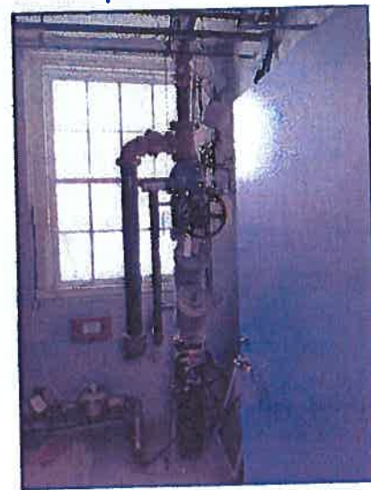
Plumbing riser for fire suppression system
