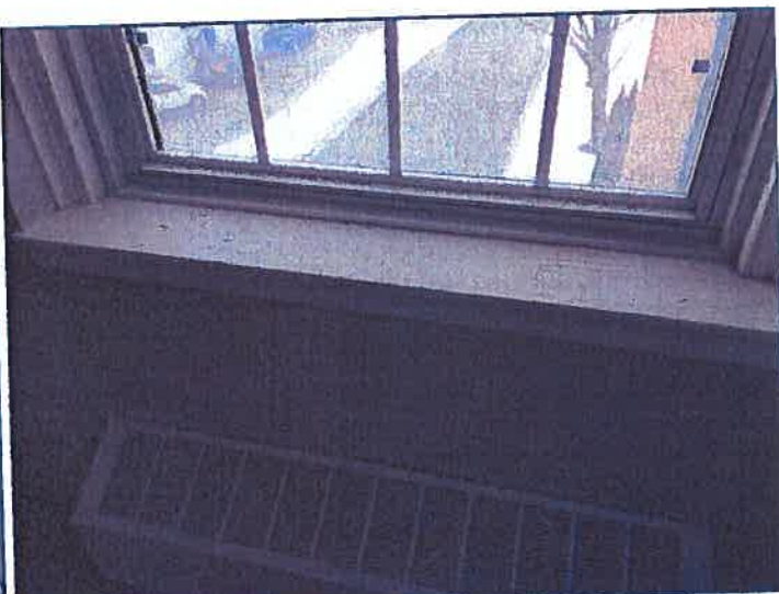
Water staining on window sills tested dry.
