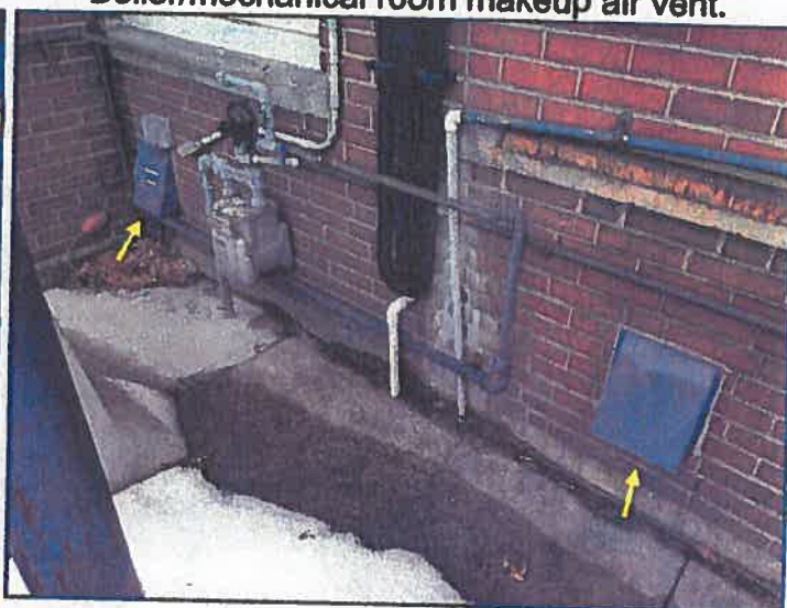
ERV vent terminations at rear of building.
