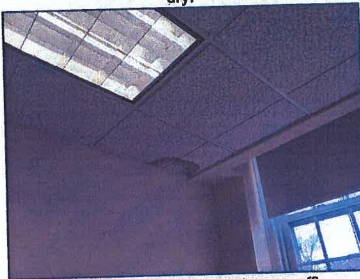
Water staining at general assistance office.
