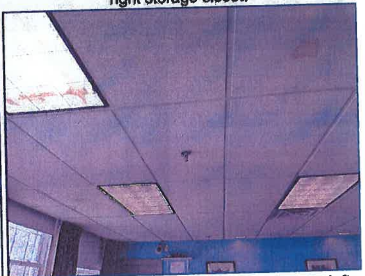
Numerous water stains at second floor rear left room / conference room ceiling.
