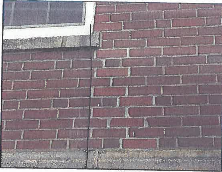
Step cracking at rear
