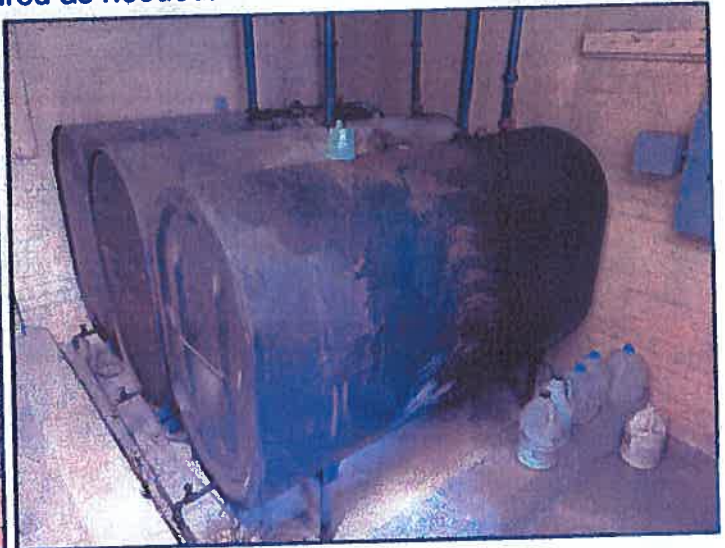
Oil staining on oil tanks
