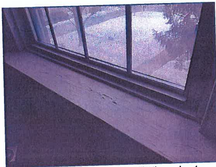
Water staining at window sills throughout.
