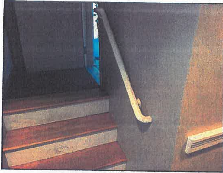
Loose railing at stage rear stairway.
