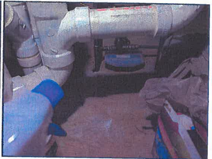
Water staining and cabinet below 3rd floor kitchen sink tested dry. Rodent activity / treatment present.
