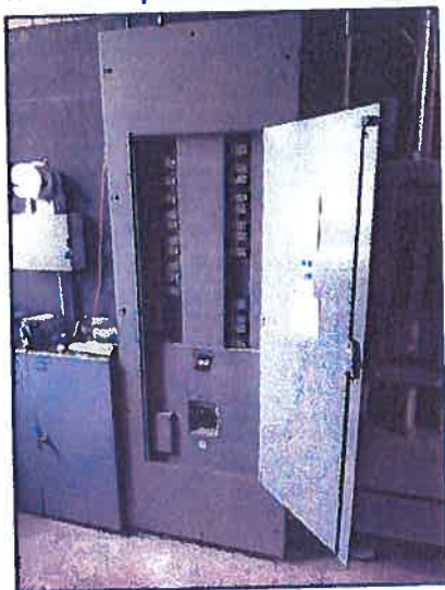
Main panel and service disconnect switch in basement mechanical room
