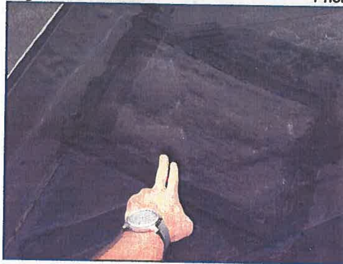
Areas of lifting at patches and seams
