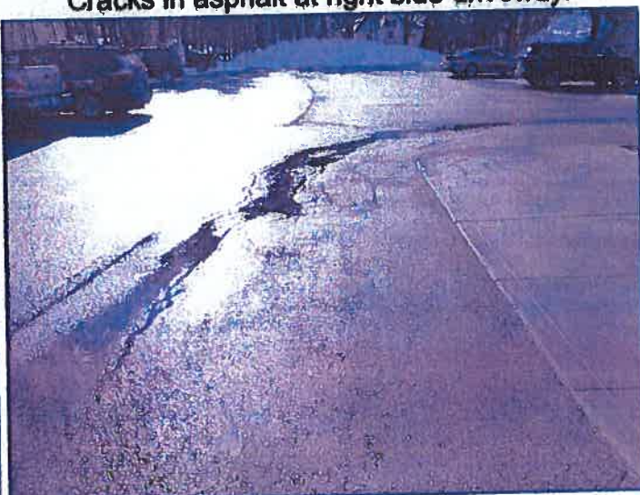
Damaged asphalt surfaces at rear building.
