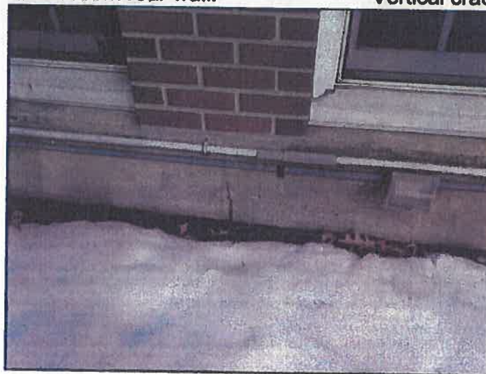
Vertical crack at front wall
