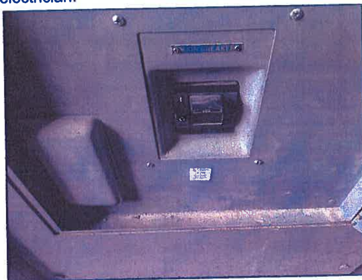
Service disconnect switch at main panel.
