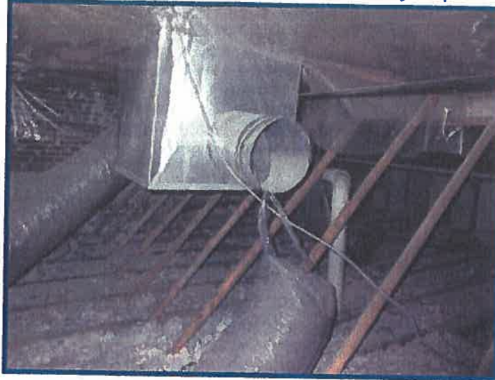
disconnected ducts in attic space
