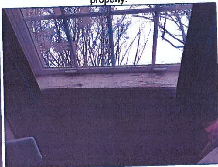
Water staining and peeling paint at many window sills.
