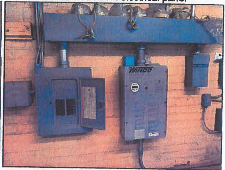
Generator automatic transfer switch and sub panel in basement mechanical room.
