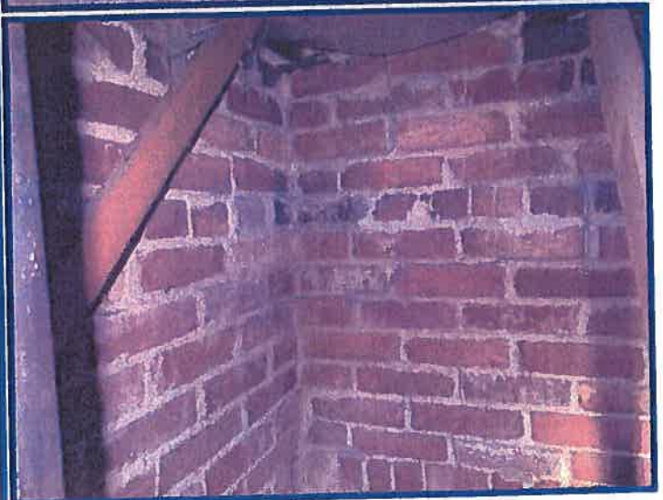
horizontal cracks and step cracks
