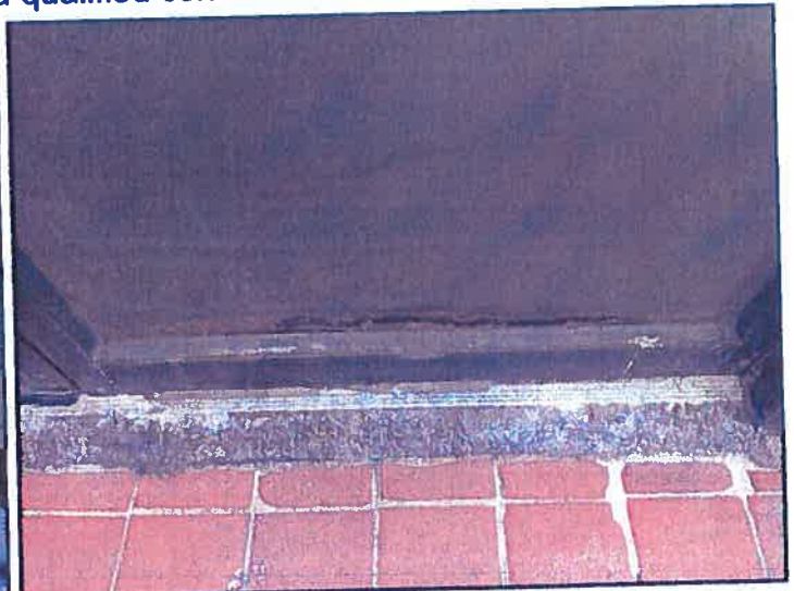
Corrosion/damage at front door
