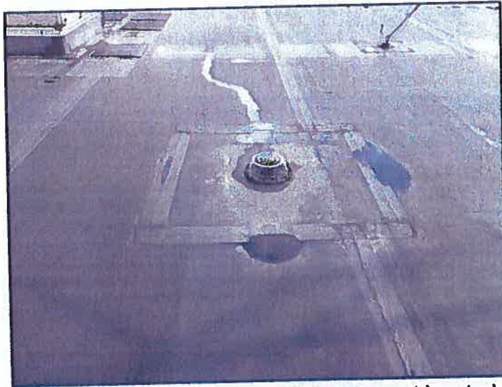
Internal roof drains. Termination was not located.
