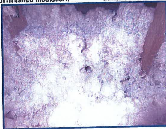
animal tunnels in insulation
