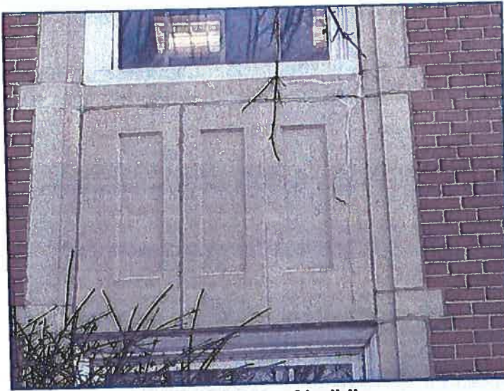
Crack at front of building
