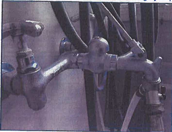
Faucet is leaking at third floor janitor closet.
