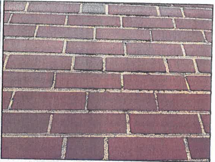
Areas of damage/receding mortar.
