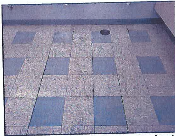
Lifting tiles / worn flooring at third floor man's room. Area tested dry.
