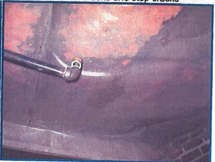
water staining above vapor barrier, dry at the time of inspection
