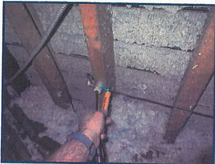
Knob and tube wiring.
