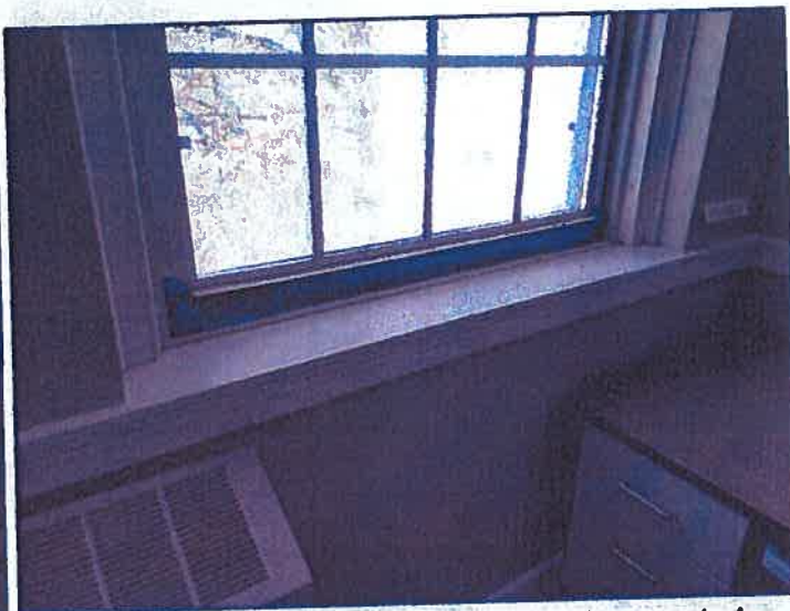
Window at third floor front left room does not close properly.
