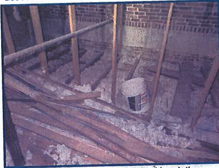
Areas of disturbed / diminished insulation.
