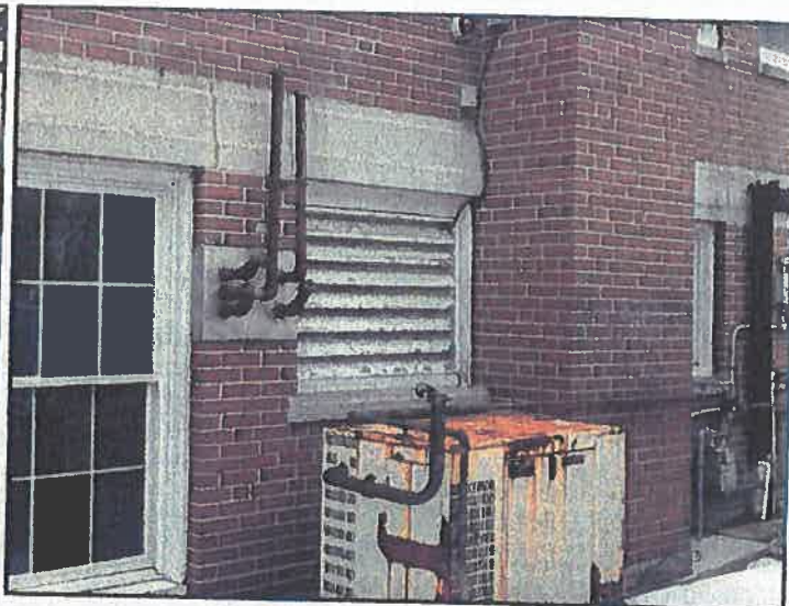
Boiler/mechanical room makeup air vent.
