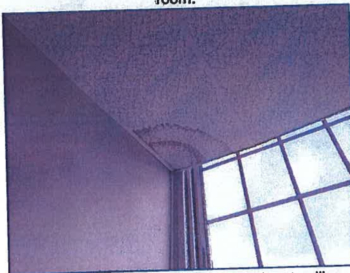
Water staining at third floor janitor closet ceiling.
