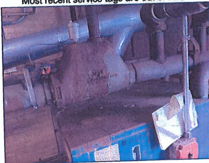
Corrosion at boiler
