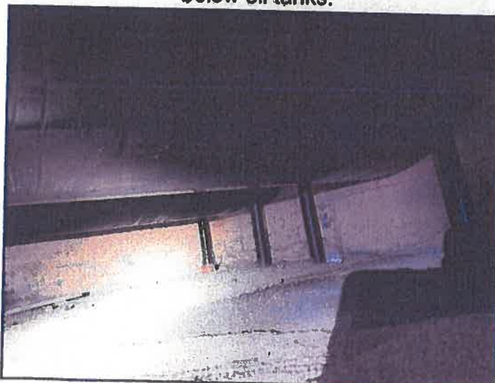
Oil leak / wet oil staining on tank and floor below oil tank.
