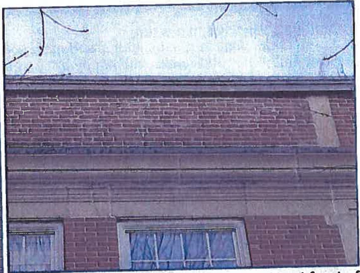
Areas of damage/deterioration to mortar at front of building.
