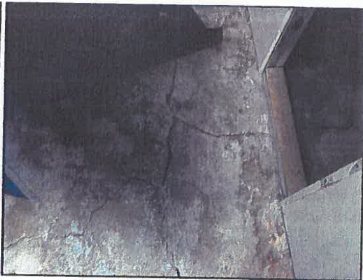
Large cracks at left side entry
