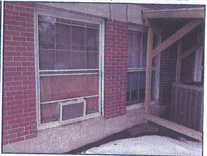
Older single pane wood windows with peeling paint and glazing
