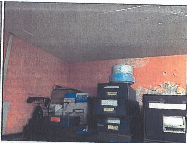
Efflorescence/water staining at vault wall.
