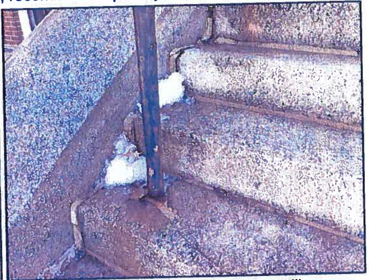
Corrosion/damage at front stair railing.
