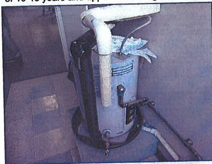
Electric water heater at third floor janitors closet, 4 years old.
