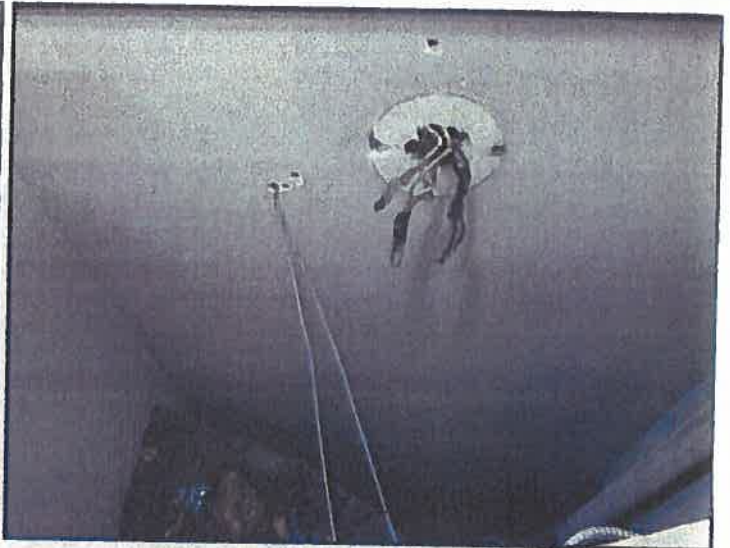
Open splice at roof access / above drop ceiling was not live at the time of inspection.
