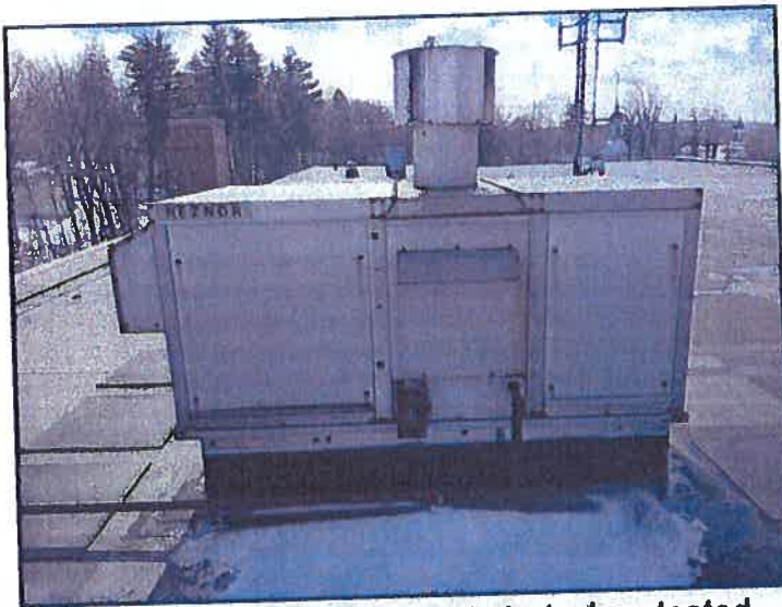
Rooftop heating unit did not start when tested. Age not determined, but unit appears to be beyond design life.
