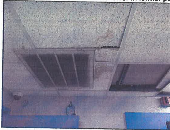
Damaged ceiling tiles and water staining at former police station. Area tested dry.
