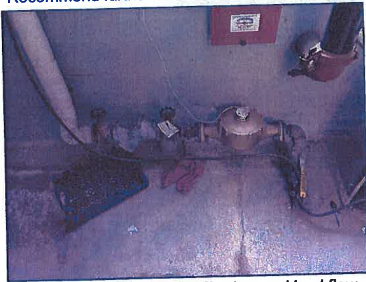
Water meter, main shut off valve, and backflow prevention device at lower level front sprinkler room.
