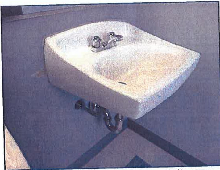
Loose sink / gap at wall at third floor ladies room. Corrosion on plumbing below sink.
