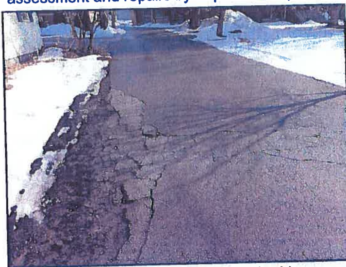
Damaged asphalt surface at left side driveway.
