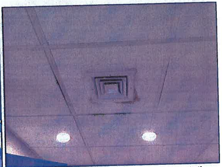
Water staining throughout former police station tested dry.
