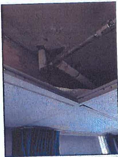
Water staining at town manager's office tested dry.
