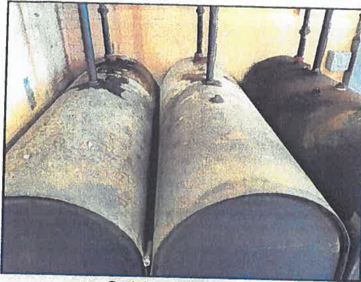
Staining on oil tanks.
