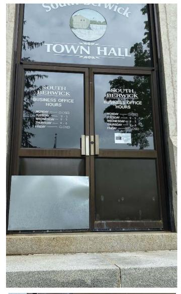
The aluminum storefront front doors are deteriorating, a panel has corroded, and the door should be replaced.
