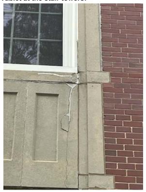
• While pieces have not fallen yet, the large cracks are allowing water into the wall / precast system, and it will continue to crack until it also fails.
