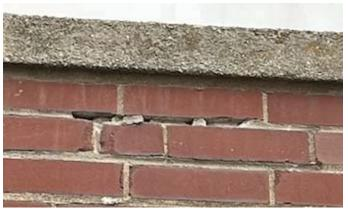
• At places, water has infiltrated the precast concrete and has started to weep through the brick causing the mortar joints to deteriorate. When the precast concrete is stabilized, any places where the mortar is failing will need repointed.
