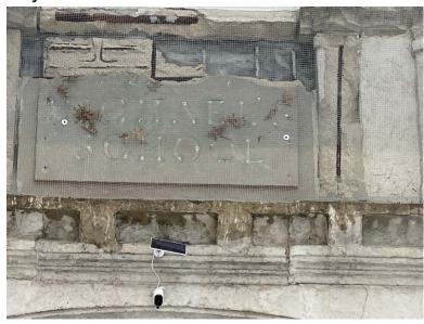
• The large piece over the main entry is in the worst shape and has totally crumbled to the point somebody has provided a protective screen around it to prevent people being hit by pieces of falling pieces of concrete. As this concrete deteriorates, it allows water into the precast and the brick wall which will accelerate the cracking of the precast and potentially the brick system.
