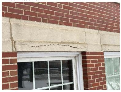
• Water has infiltrated the window header in several places and the rebar has started to rust and expand creating a long, continuous crack. This situation will continue to get worse unless some sort of remediation is done.
