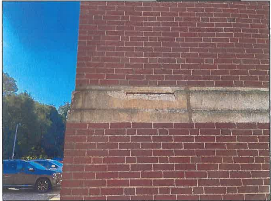
Photograph 1 – Concrete Banding Deterioration
