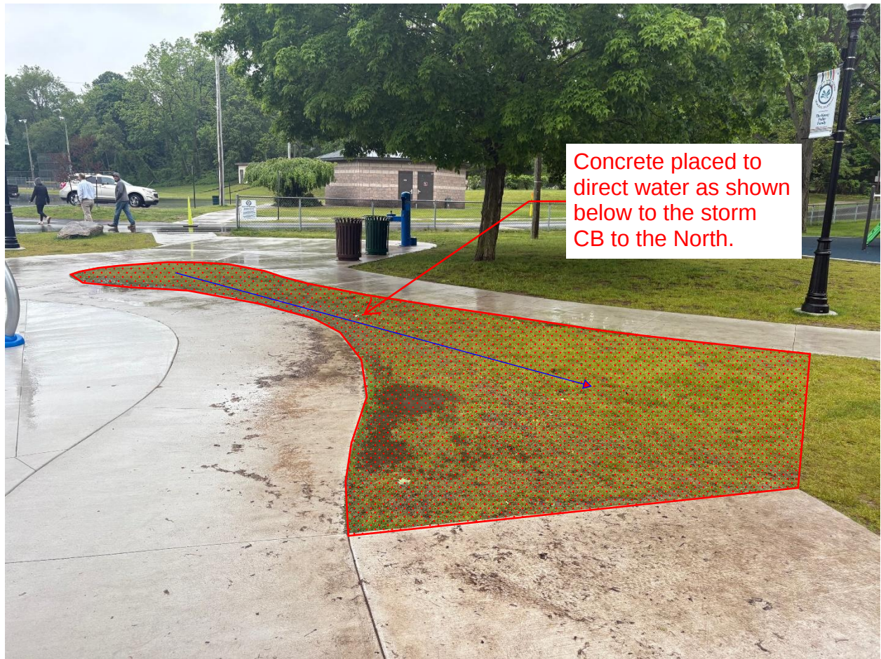
Area 1: Approx 506 SF of 4" exterior concrete
