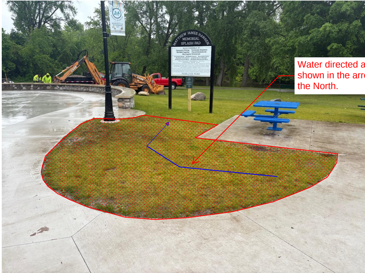
Area 2; Approx 314 SF of 4" exterior concrete
