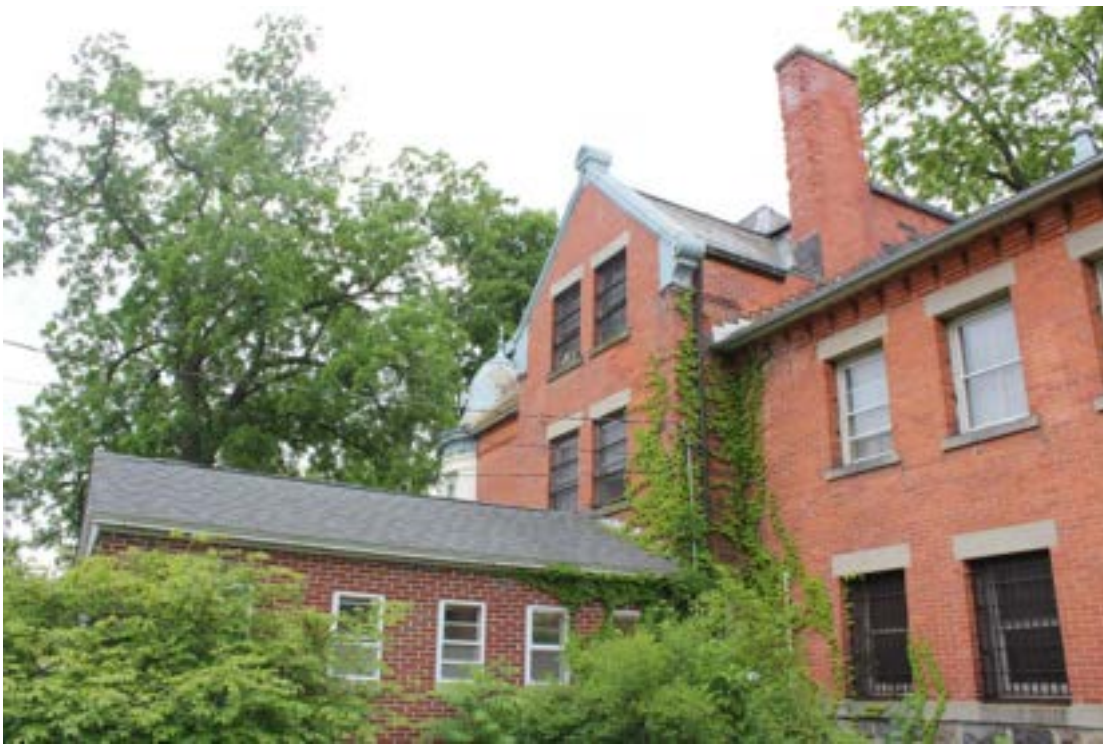
Image 18 Looking east at the 1959 addition located at the center section of the north elevation. This addition has an asphalt-shingled roof with vegetation growing against the flashing and valleys of the roof where the addition adjoins the sheriff's residence. Ivy has spread across the lower and upper stories of this
