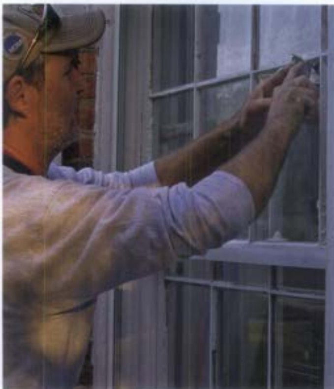
Figure 11. Glazing putty should be maintained in sound condition to prevent unwanted air infiltration and water damage. New glazing putty should be pulled tight to the glass and edge of the wood, creating a clean bevel that matches the historic glazing.
