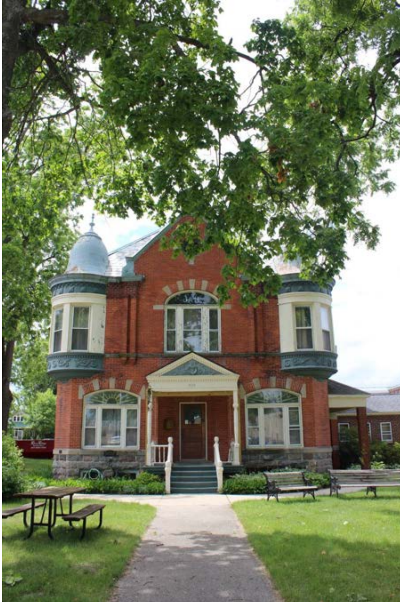
Image 3 Head-on view of the old jail's façade, looking west. Vegetation is growing in areas against the foundation at grade. Vegetation brings moisture against the rock and grows against mortar which accelerates deterioration.
