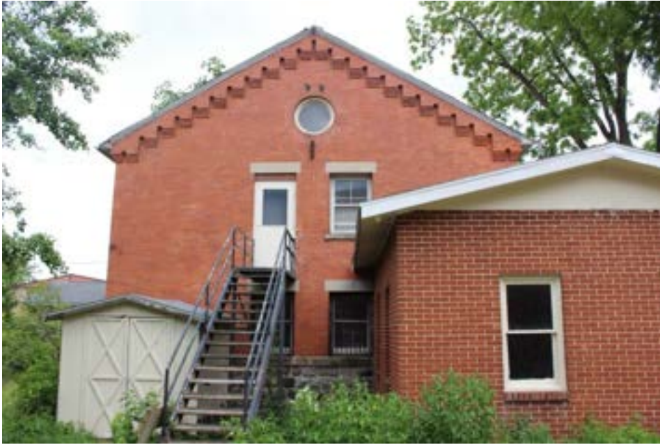
Image 16 Direct view of the jailhouse's west elevation, looking east. There's a significant amount of vegetation against the rear of the structure. Overall, the masonry at this elevation looks to be in good condition. A small shed is located at the northwest corner of the west elevation.
