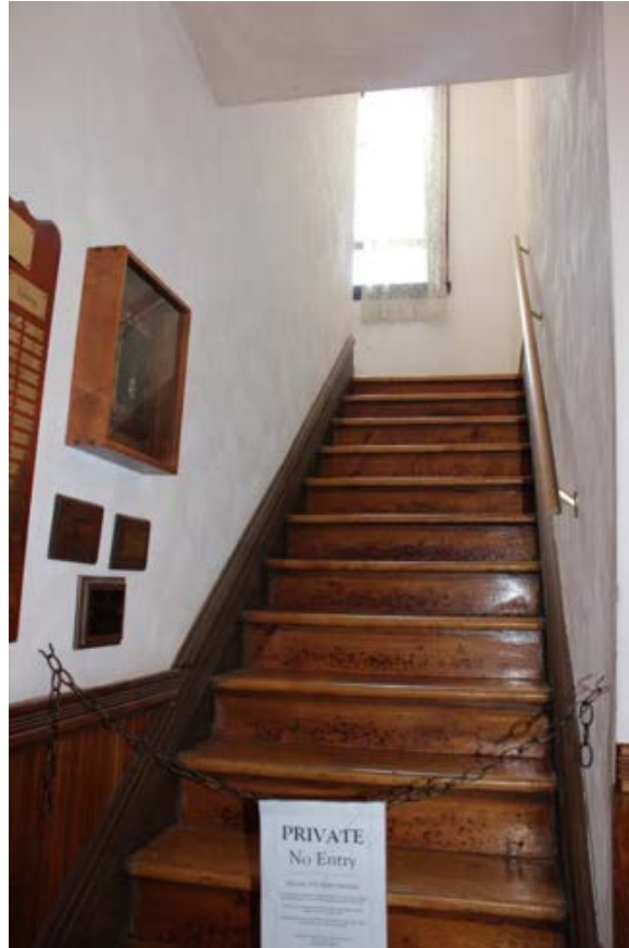
Image 27 Looking north at the stairs that lead to the upper floors of the sheriff's residence. Wood floors, trim, molding, and plaster are all in good condition in this area.
