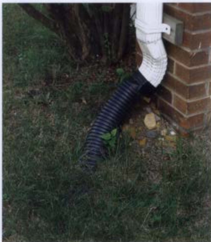
Figure 17. Extending downspouts at their base is one of the basic steps to reduce dampness in basements, crawl spaces and around foundations. Extensions should be buried, if possible, for aesthetics, ease of lawn care, and to avoid creating a tripping hazard. Photo: NPS files.
