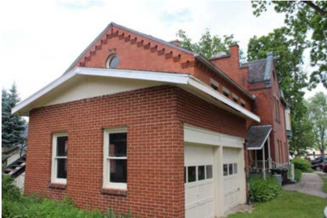
Image 15 Oblique view of circa 1930s garage addition. This addition is adjacent (attached) to the 1893 kit jailhouse which is directly west of the main sheriff's residence that was constructed in 1897. Two, one-over-one windows are located at the west elevation of the garage with side-gabled roof.
