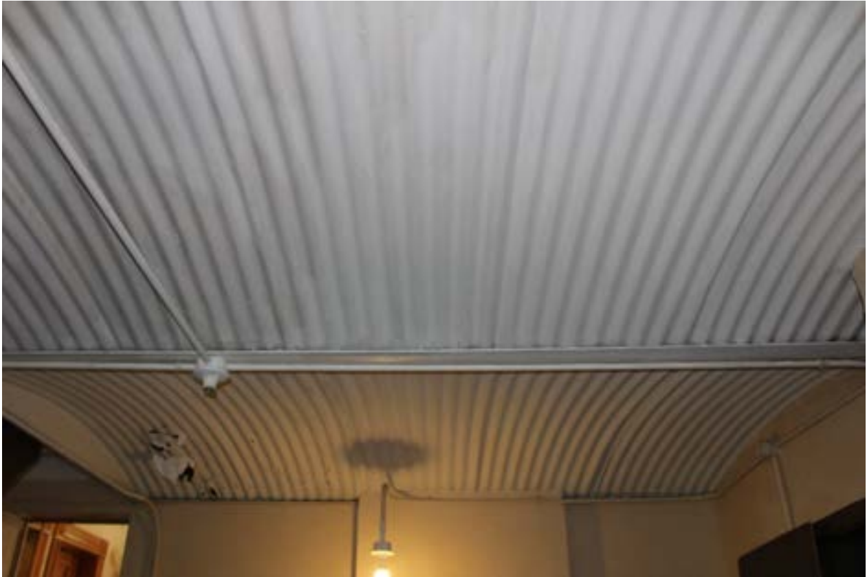
Image 34 Looking south at the ceiling detail in the room adjacent to the kitchen and the jail cells. This ceiling is like a Quonset hut shape with corrugated metal.
