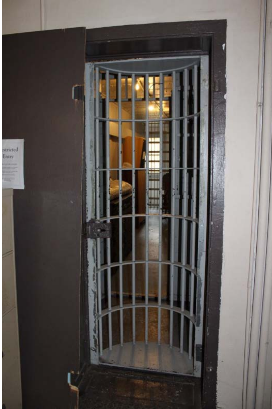
Image 30 Looking north in the jail cell section of the jail kit house. All original jail cells are intact with operable mechanisms.
