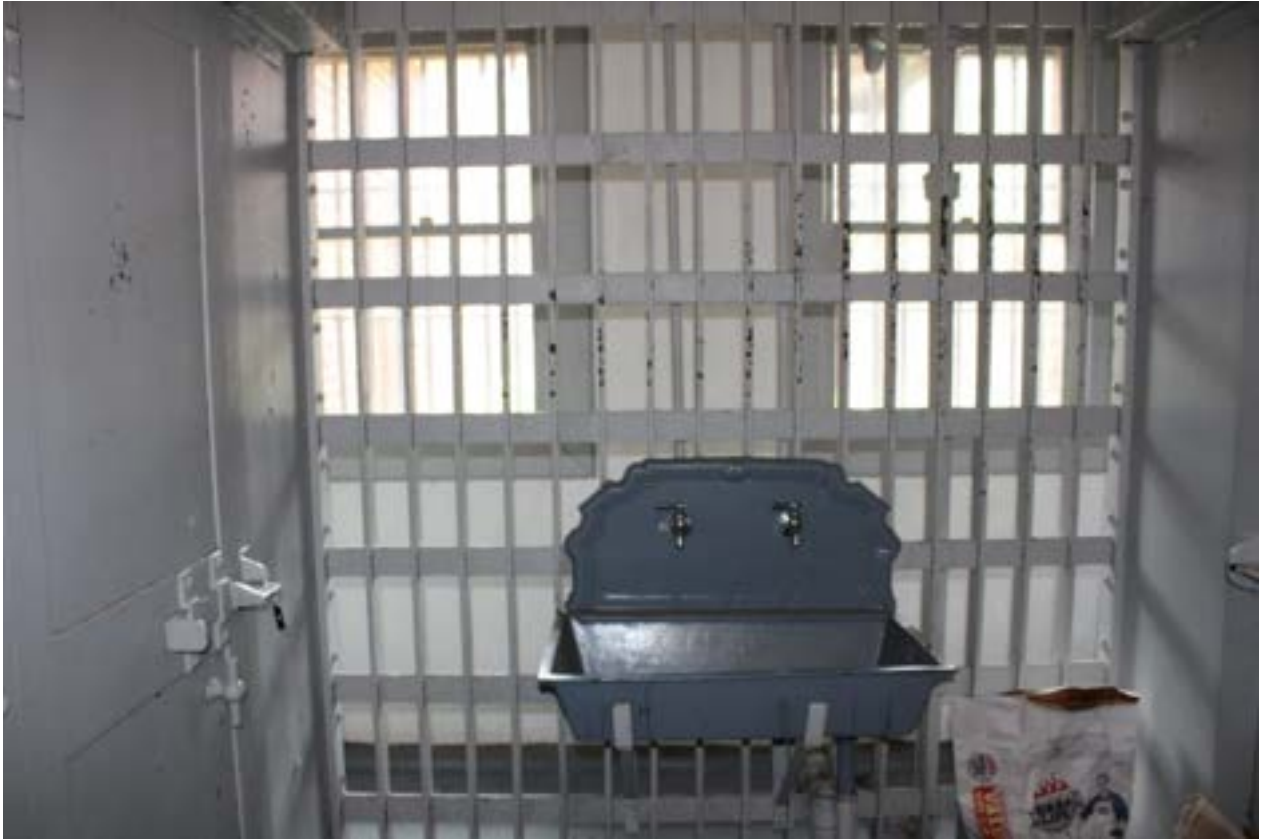
Image 31 Looking south in a jail cell at the original sink.
