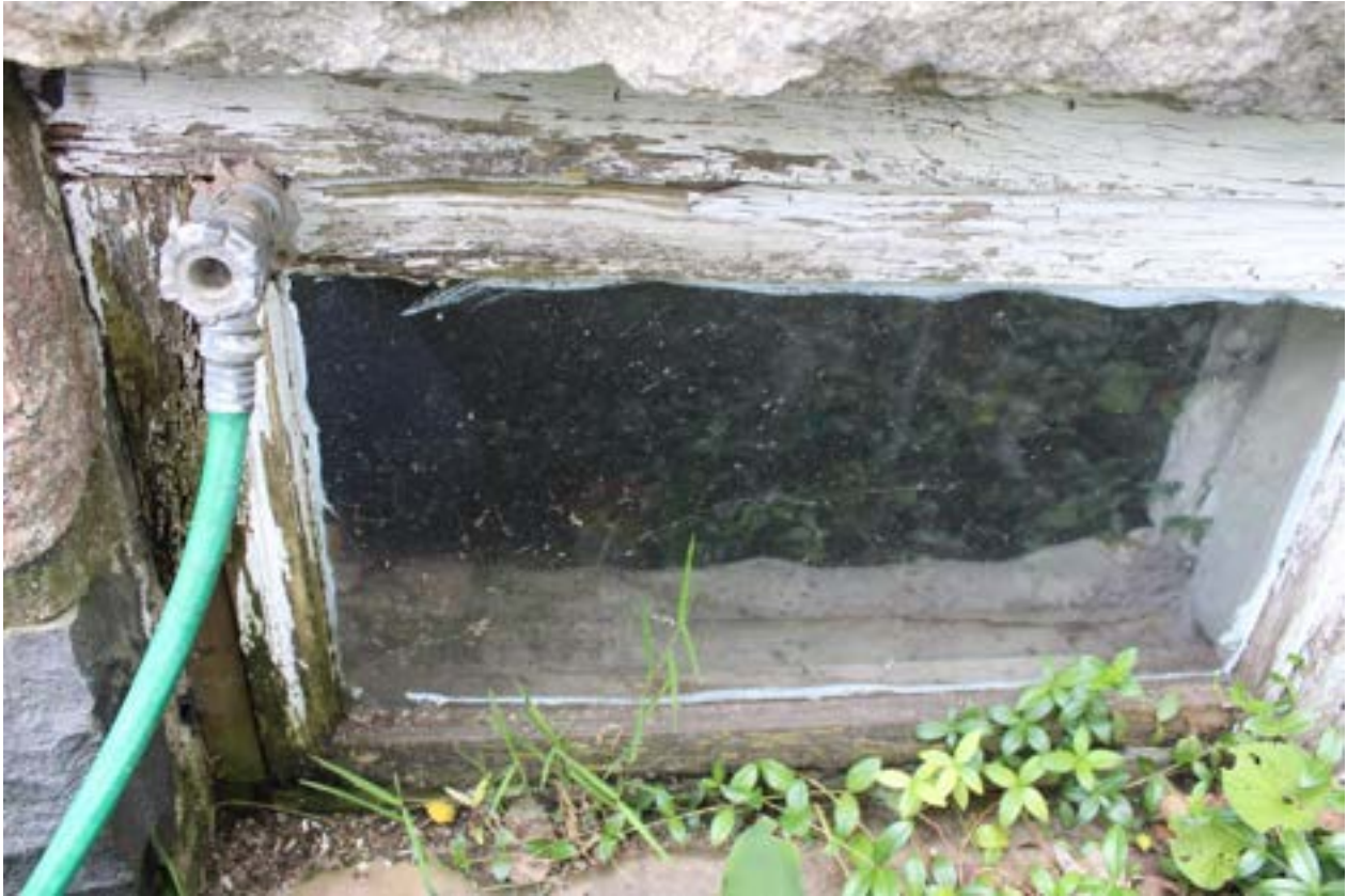
Image 14 Rectangular window to raised basement on south side of façade at the foundation level, looking west. Visible water damage and wood rot. Water could be coming off the hose which is installed against the window sash/casing, because of vegetation against the window, or a combination of both.
