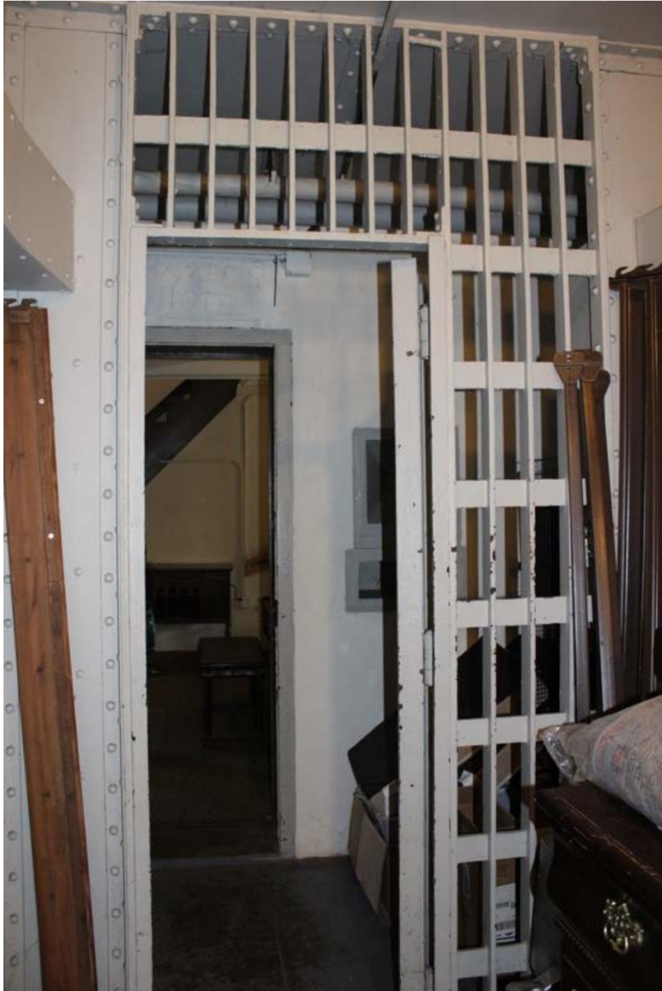
Image 33 Looking east in the entrance to the jail cells at the room just off the kitchen.
