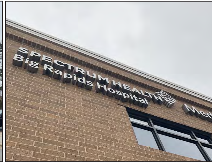
Existing - Image 3 (Angled View)
