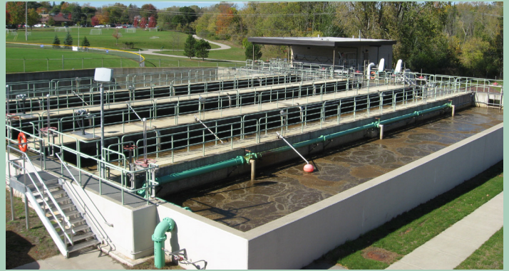
Aeration basins at the Wastewater Treatment Plant.
