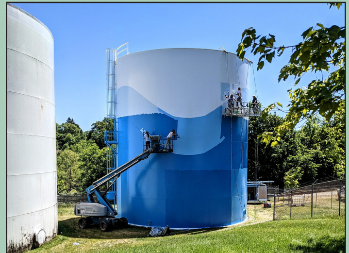
Water Plant reservoirs being repainted.
