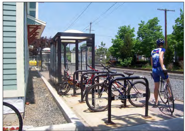
This multi-modal station provides commuter rail access, bus access, and bicycle parking
