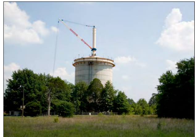
The new City of Columbia water tower off of Rimer Pond Road is now completed
