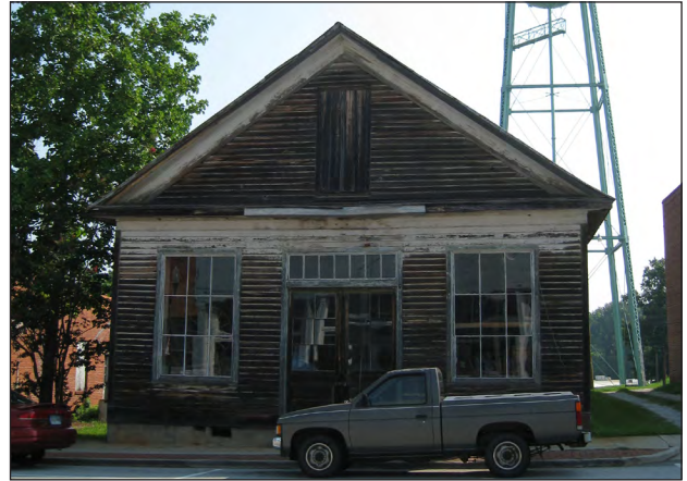
The nearby town of Ridgeway includes this Greek revival commercial building
