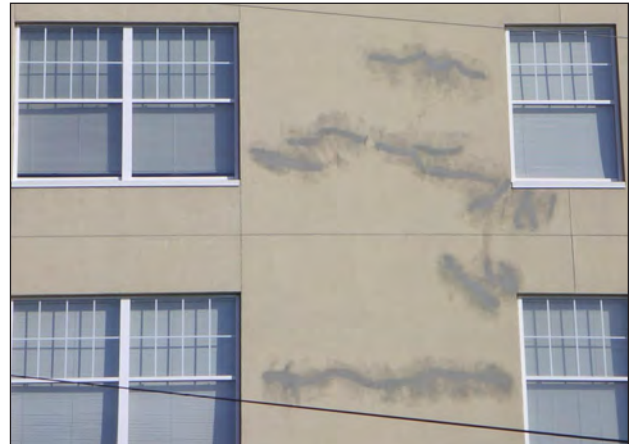
Exterior insulation finishing systems (EIFS) are not acceptable, for aesthetic reasons and short lifetime
