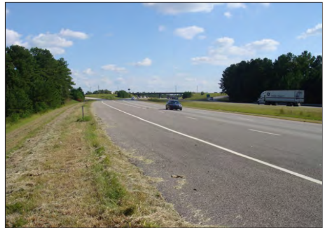
Interstate 77 presents a barrier to street connectivity within the town, particularly for non-automotive travel
