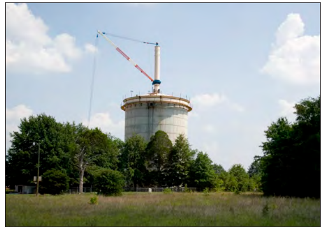
Public water provided by the town could be a source of revenue and help guide redevelopment
