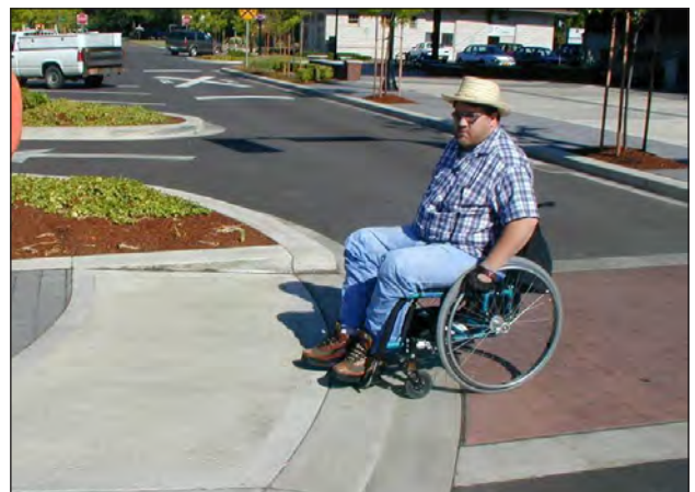
Sidewalks and crosswalks must comply with the Americans with Disabilities Act (courtesy Michael Ronkin)
