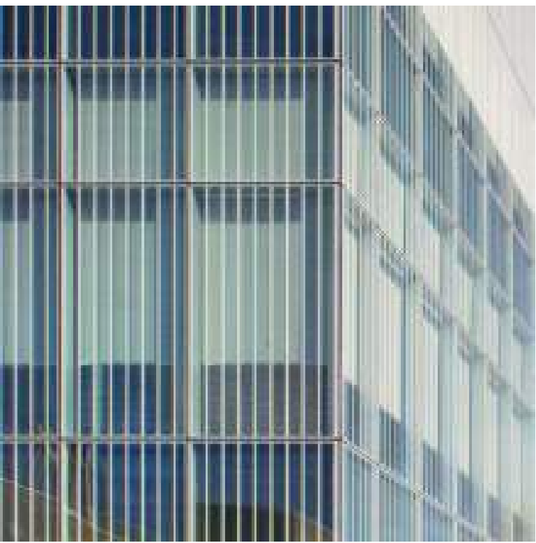
SOLID OR FRITTED PANELS, GLAZED INTO CURTAINWALL
