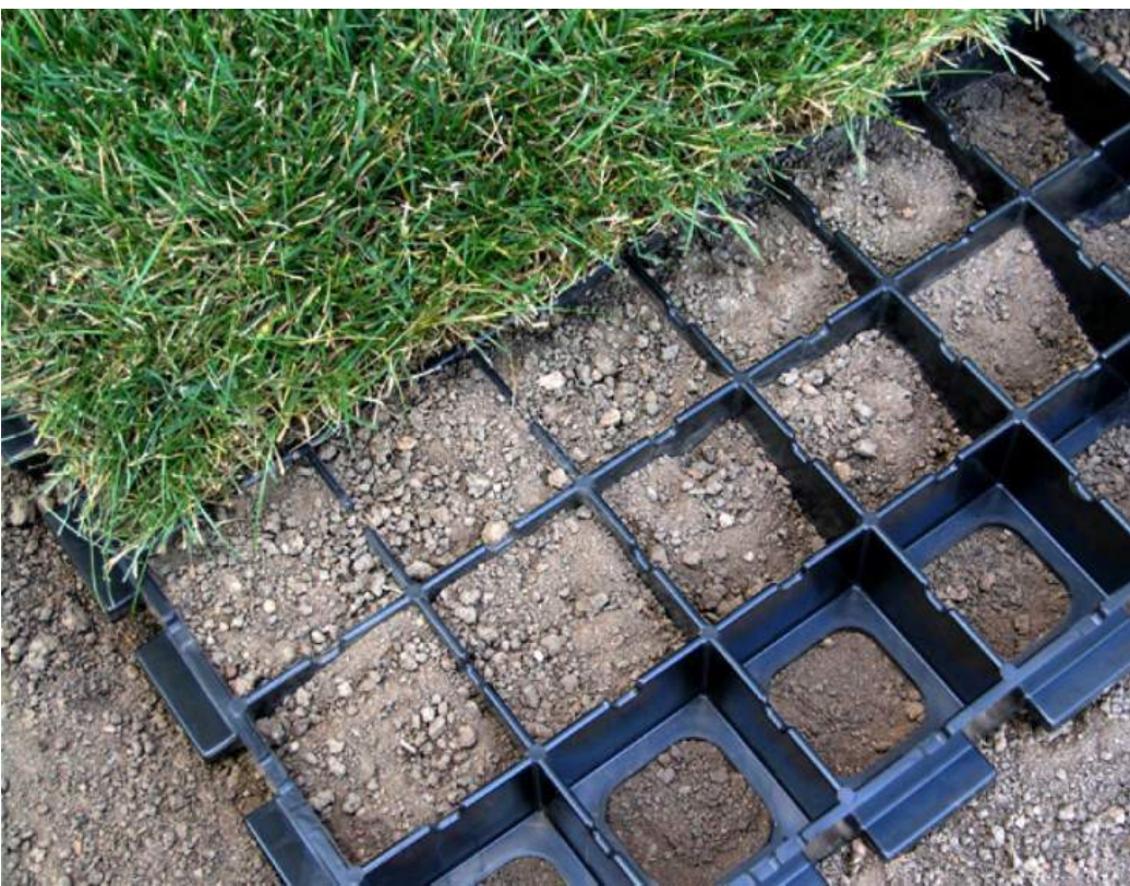
REINFORCED GEOBLOCK PAVING SURFACE - LIMITED USE AT EMERGENCY VEHICLE ACCESS LANES
