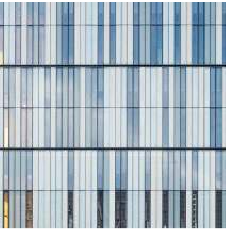
SOLID OR FRITTED PANELS, GLAZED INTO CURTAINWALL
