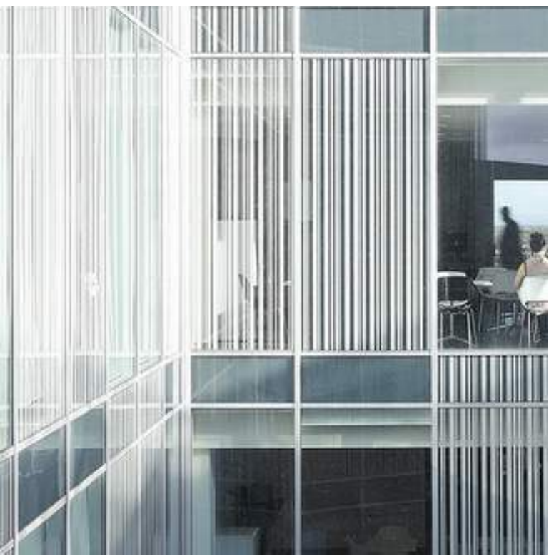
SOLID OR FRITTED PANELS, GLAZED INTO CURTAINWALL
