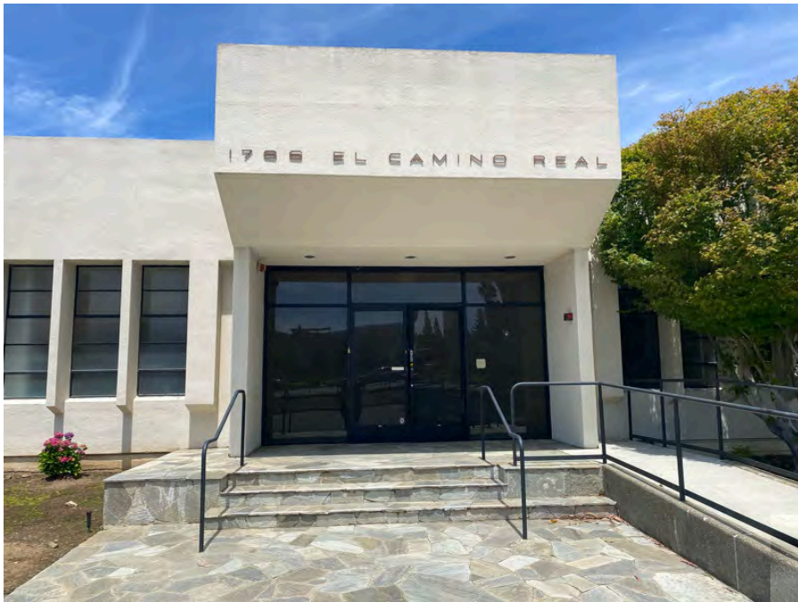
Photo 2: View looking north at the subject property.
