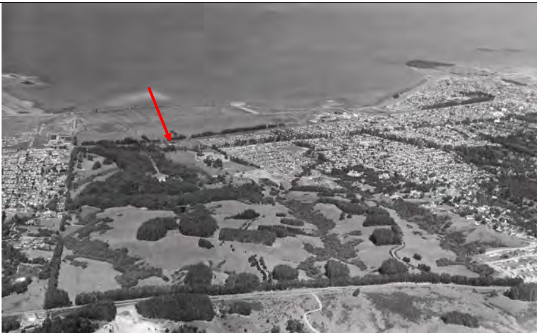
Figure 10: Aerial photograph of the Darius Ogden Mills Estate, date unknown. The red arrow points to the approximate location of 1766 El Camino Real, constructed in 1959.
