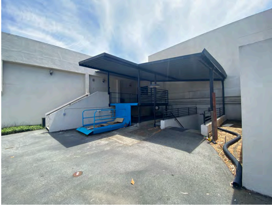
Photo 7: View looking south at the subject property.
