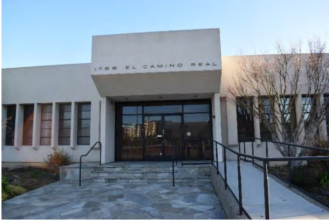
Figure 2. View of west façade, facing east. Source: ICF 2/12/2020.
