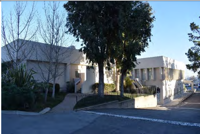
Figure 4. View of south façade, facing northeast. Source: ICF 2/12/2020.
