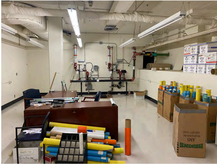
Photo 9: View looking at the interior of the subject property.
