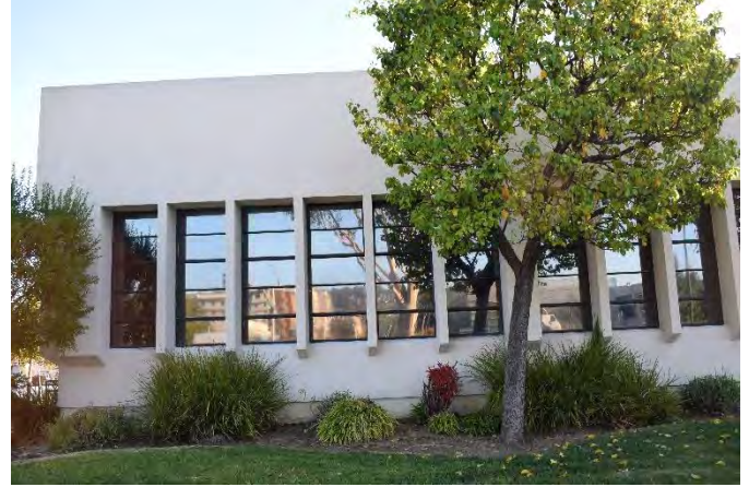
Figure 3. View of west façade, facing east. Source: ICF 2/12/2020.
