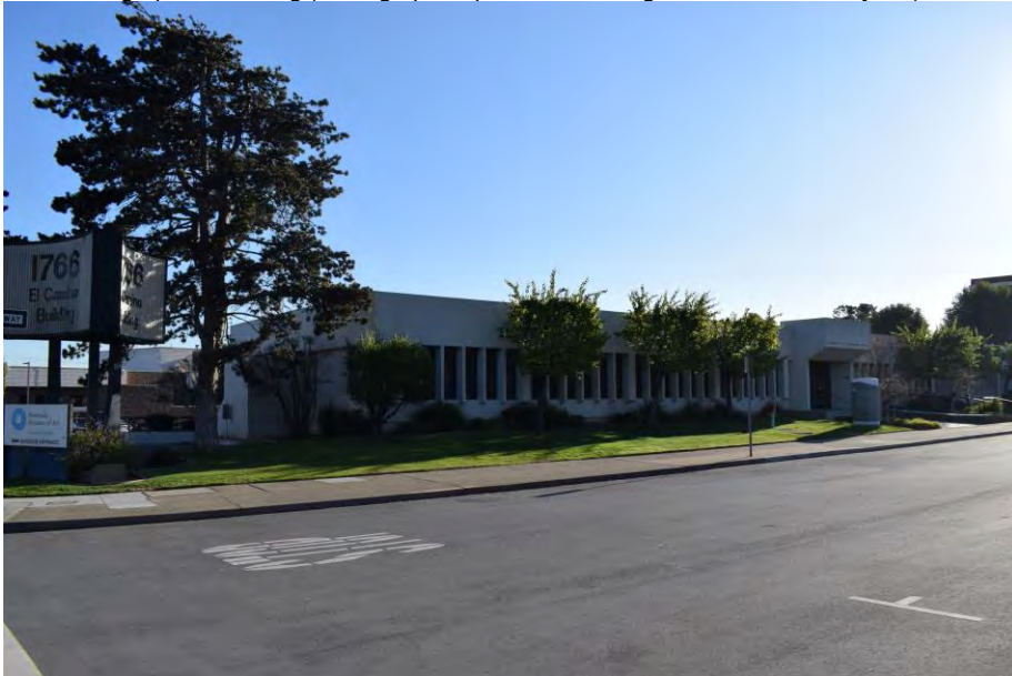
Figure 1: View of north and primary (west) façades, facing southeast. Source: ICF, 2/12/2020.
