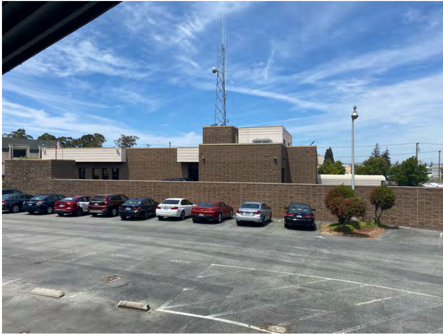
Photo 15: View looking north at the adjoining property to the north.
