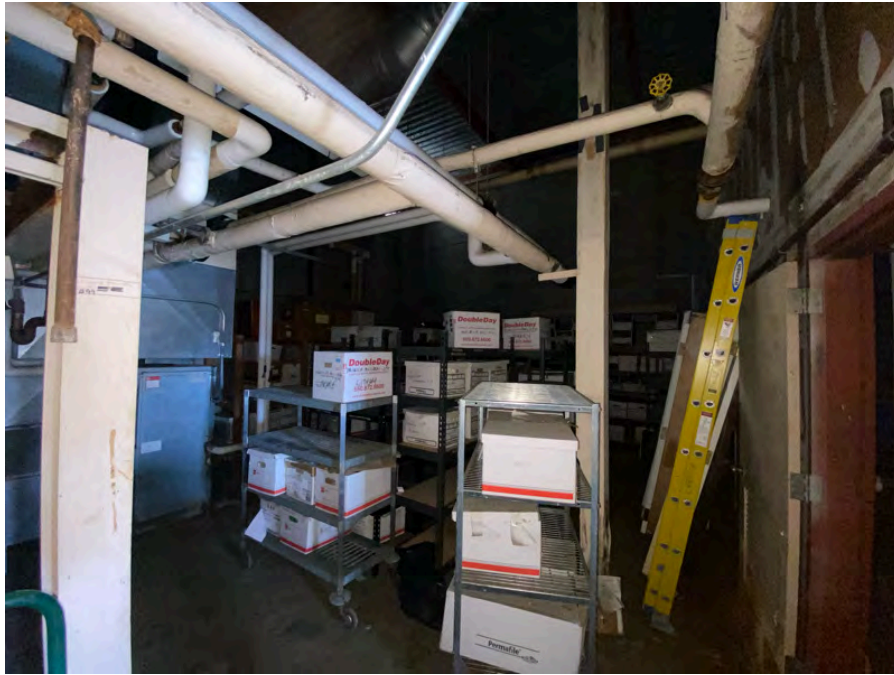
Photo 11: View looking at the interior of the subject property.
