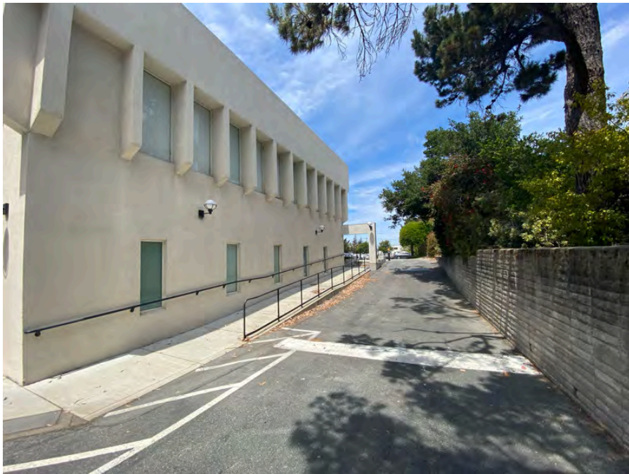
Photo 4: View looking north at the subject property.
