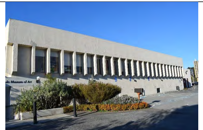
Figure 7. View of the east façade, facing west. Source: ICF 2/12/2020.
