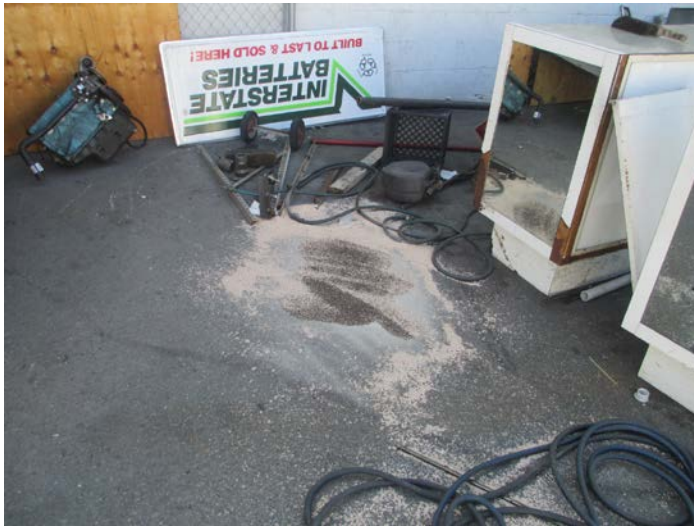
9. View of oil staining on asphalt with absorbents applied.
