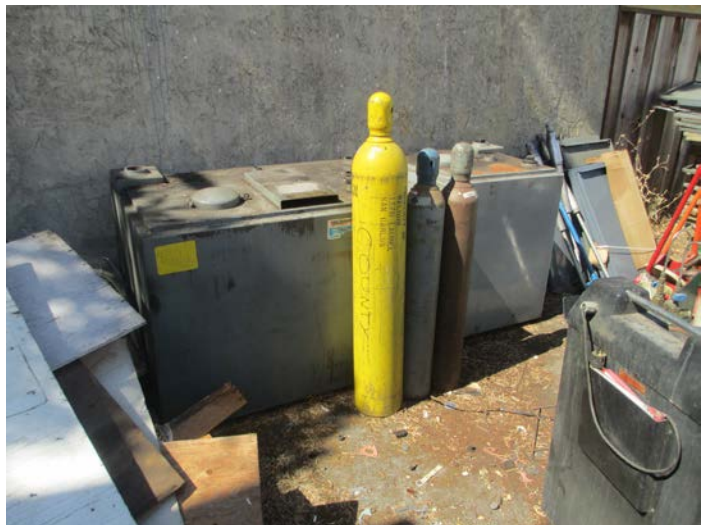
4. View of two new oil ASTs and compressed gases.
