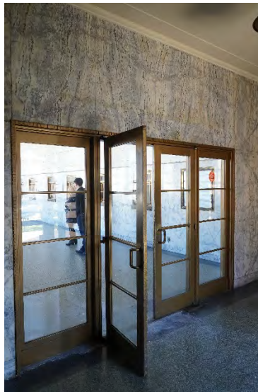
Figure 6: Vestibule doors to lobby.
