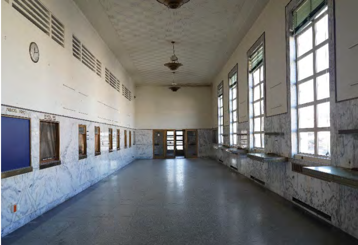
Figure 3: Lobby, looking towards the Park Road entrance.
