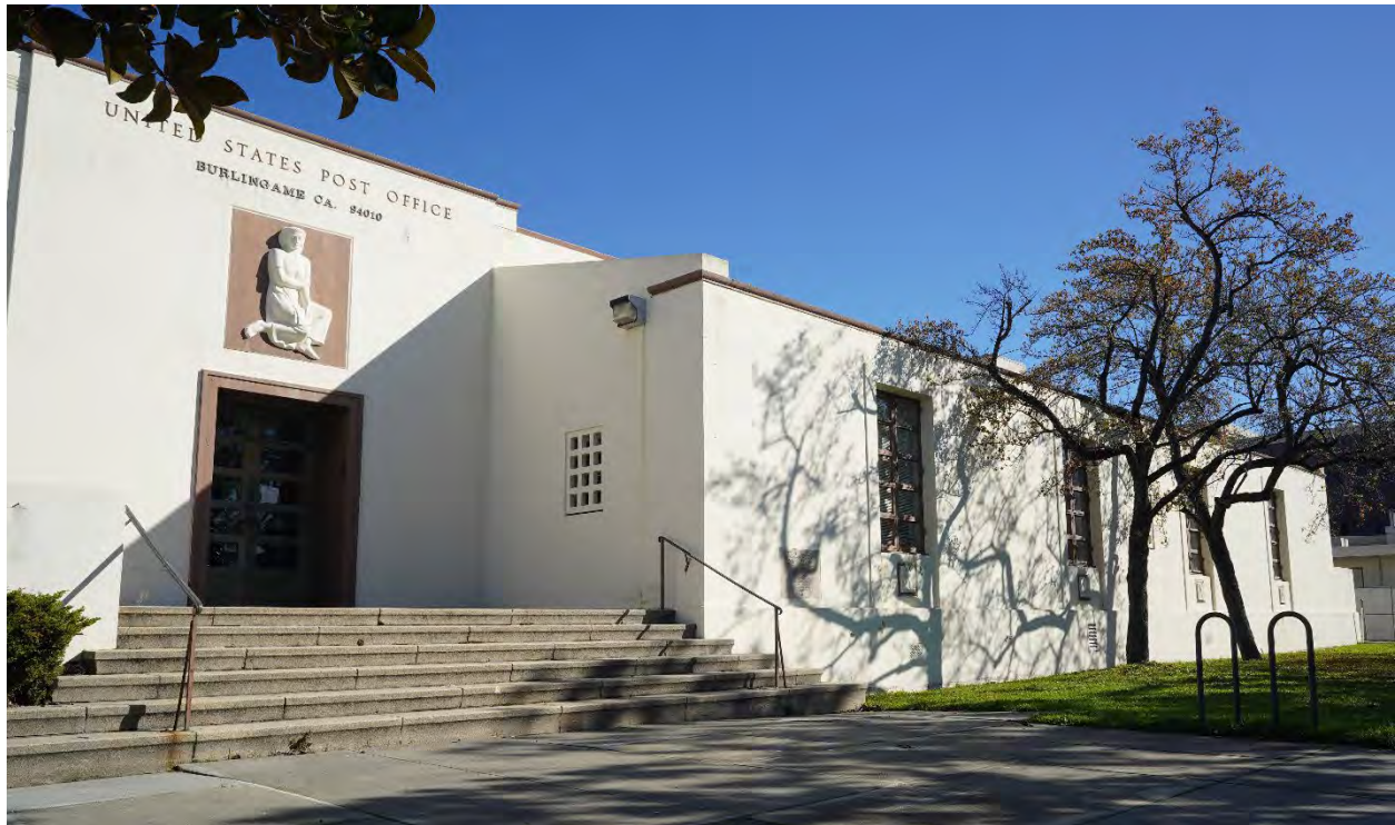
Figure 2: Park Road (southwest) façade, looking northeast.
