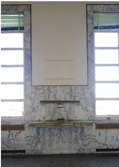
Figure 5: Cantilevered desks between lobby windows.
