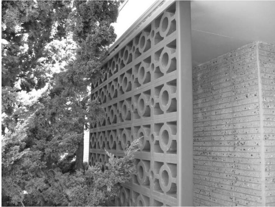
Photo 3: View of reinforced concrete screen on front façade.
