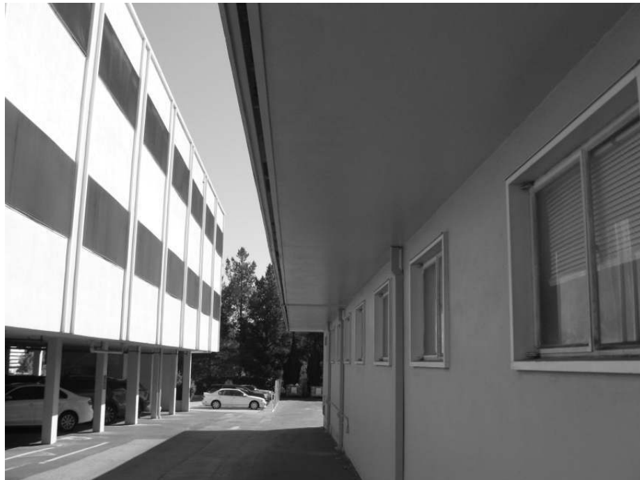
Photo 6: View along the northern façade showing cantilevered eaves.
