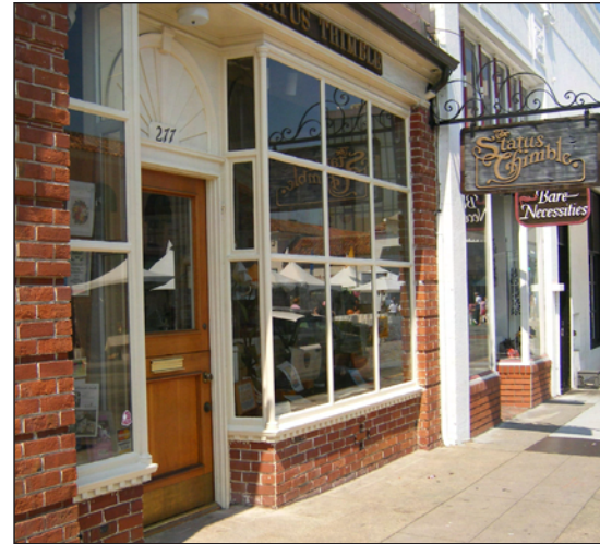
FIGURE 5-14: Size, division and shape of display windows should maintain the established rhythm of the streetscape
