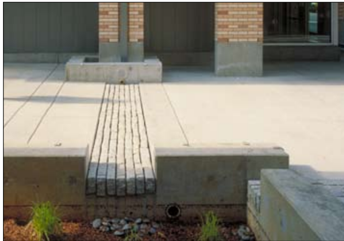
Bio-retention basins, bioswales, and detention basins can assist in stormwater retention and treatment where there is sufficient site area.
