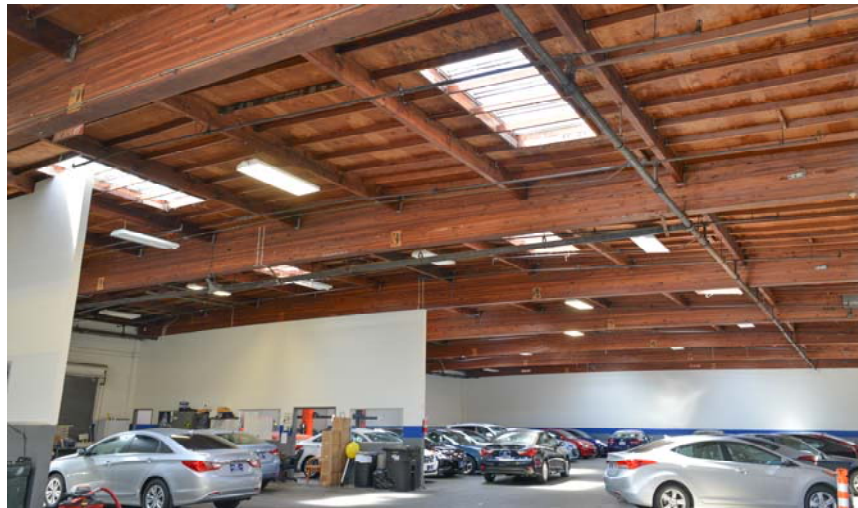
Figure 13. Glue-laminated beams in the later addition at 1025 Rollins Road.
