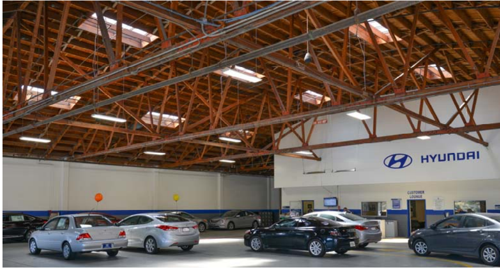
Figure 12. Bowstring trusses on the interior of the earlier addition at 1025 Rollins Road.
