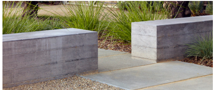
concrete seatwalls - poured in place
