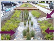
Rocks slow the flow of water as it enters the area. This prevents soil erosion by dispersing the water evenly upon entry.
