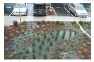
Bioretention areas function as soil and plantbased filtration devices that remove pollutants through a variety of physical, biological, and chemical treatment processes. These facilities normally consist of a ponding area, mulch layer, vegetation and biotreatment soil mix.
